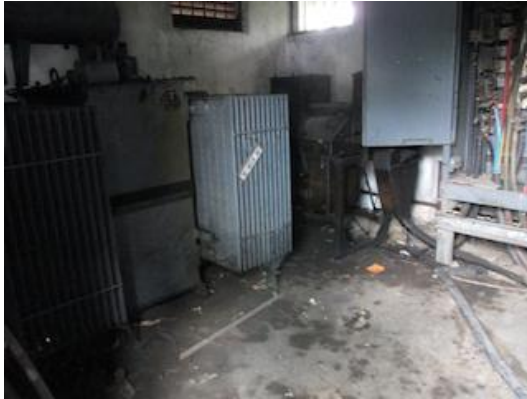
Photo 6. A substation in Yangon to be rehabilitated. Note the traces of oil spill around the transformer area.
