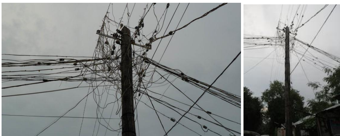
Photo 1. Wooden poles and distribution lines to be replaced with concrete poles
