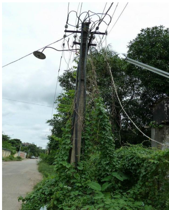
Photo 9. Vegetation growth on an electric pole.
