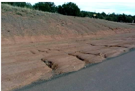
Figure 7c: Erosion of fill slope
