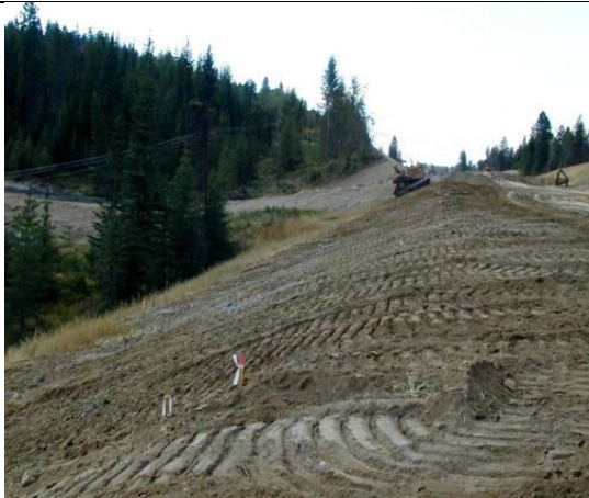
Figure 7i: Raw Graded fill slope
