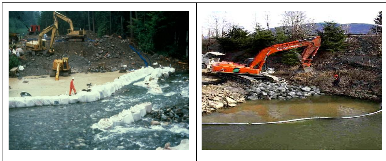
Figure 10: Examples of On-Site Mitigation Measures: Use of gravel-filled bags and plastic to isolate the work area or a boom and silt curtain
