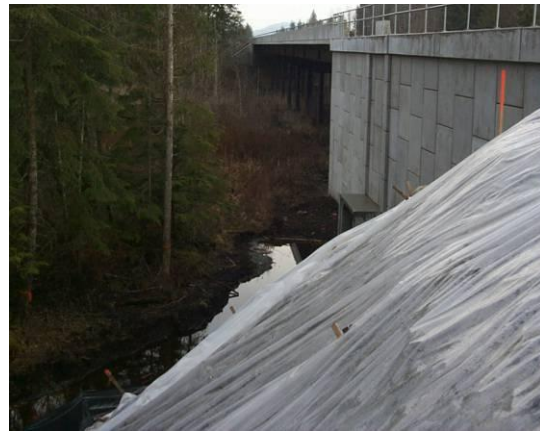
Figure 7h: Using .12mm plastic sheeting to prevent erosion
