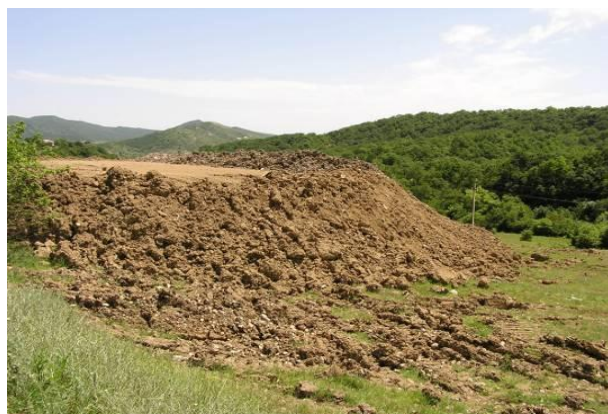
Figure 8a: How not to stockpile
