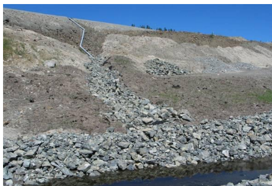
Figure 7d: Using rock to stabilize fill slope
