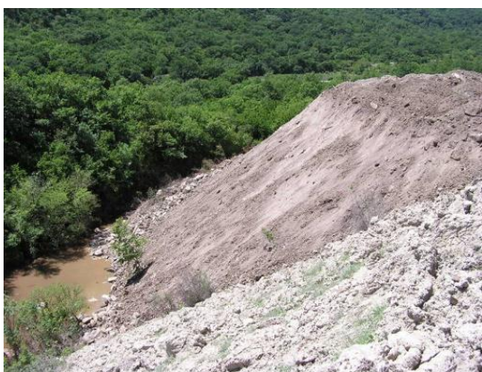
Figure 7e: Unstable fill slope
