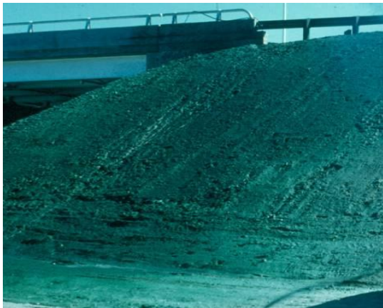
Figure 7g: Unprotected bridge end-fill
