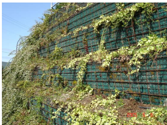
Figure 7b: Slope benched and stabilized with vegetation
