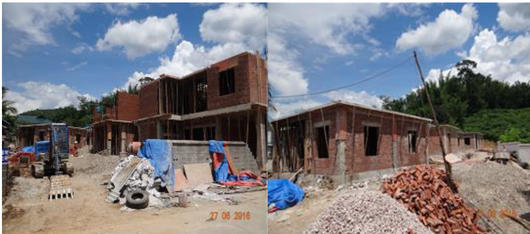
Figure 3-4 Construction Site of the Manglian Resettlement Site for Paliang Village
