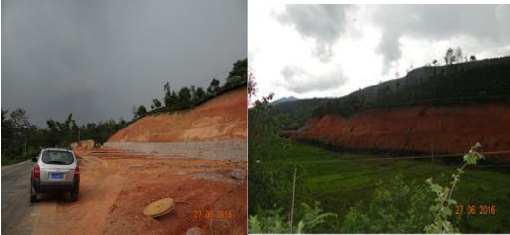
Figure 3-3 Construction Site of the Resettlement Site for Yintai Groups 1 and 2 of Paliang Village
