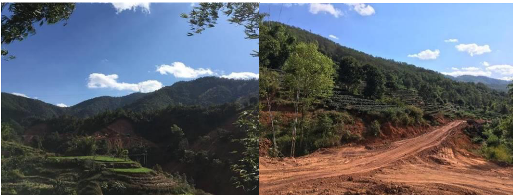
Attached Figure 2-7 Construction site with slope protection removed
