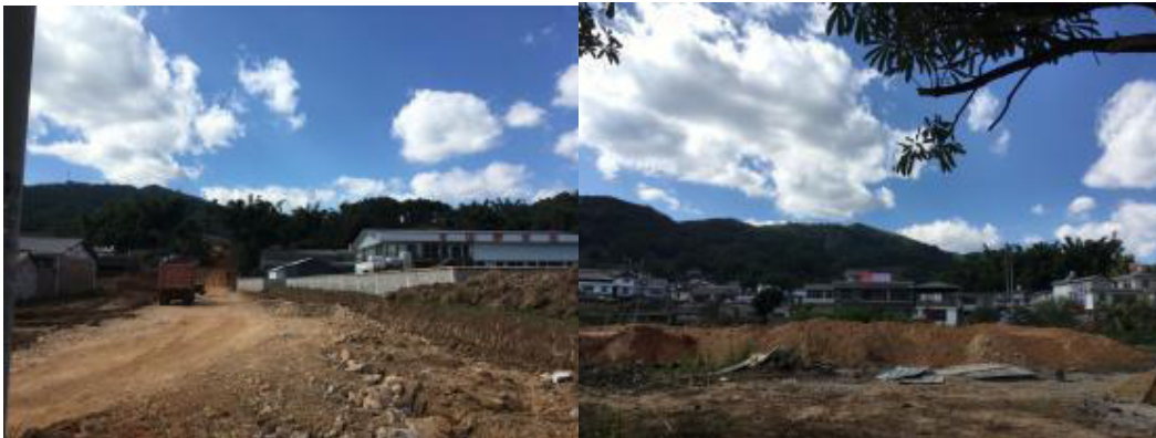
Attached Figure 2-5 Site of rerouted Ning'er Avenue
