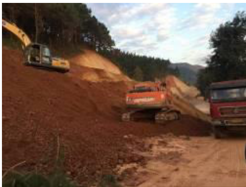
Construction site of Contract 7 in Ning'er Town
