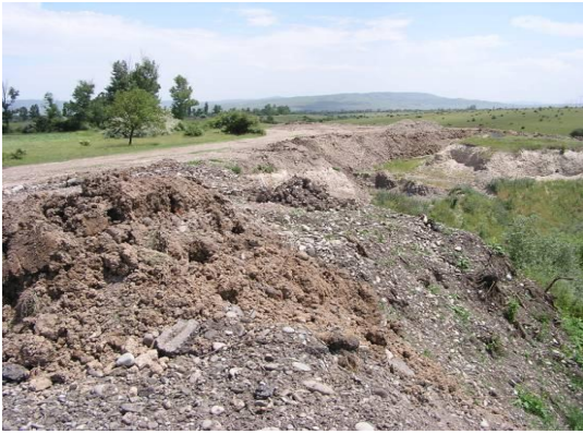
Figure 7a: Slope failure
