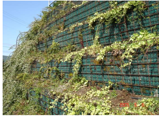
Figure 7b: Slope benched and stabilized with vegetation
