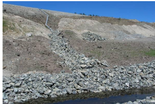
Figure 7d: Using rock to stabilize fill slope
