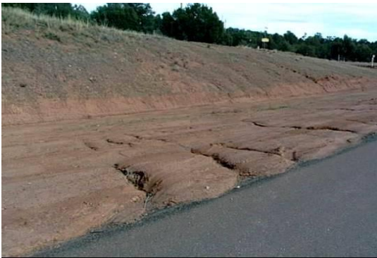
Figure 7c: Erosion of fill slope
