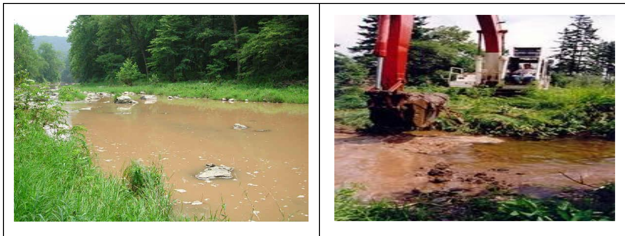
Figure 9: Examples of Unacceptable Levels of Sedimentation without Mitigation Measures
