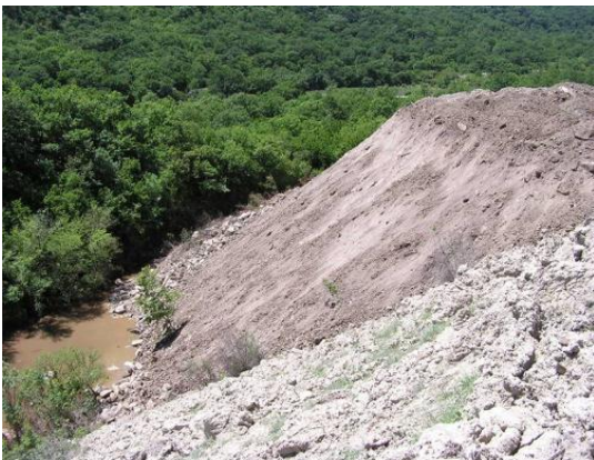
Figure 7e: Unstable fill slope
