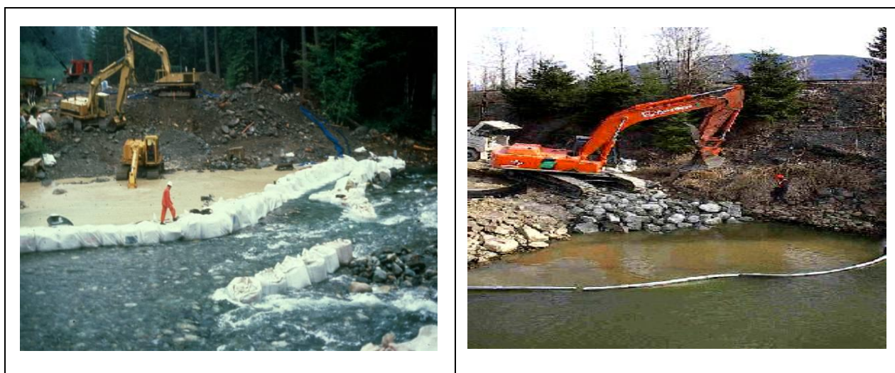
Figure 10: Examples of On-Site Mitigation Measures: Use of gravel-filled bags and plastic to isolate the work area or a boom and silt curtain
