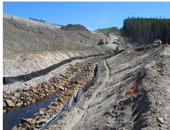
Figure 7f: Using silt fence to mitigate slope erosion
