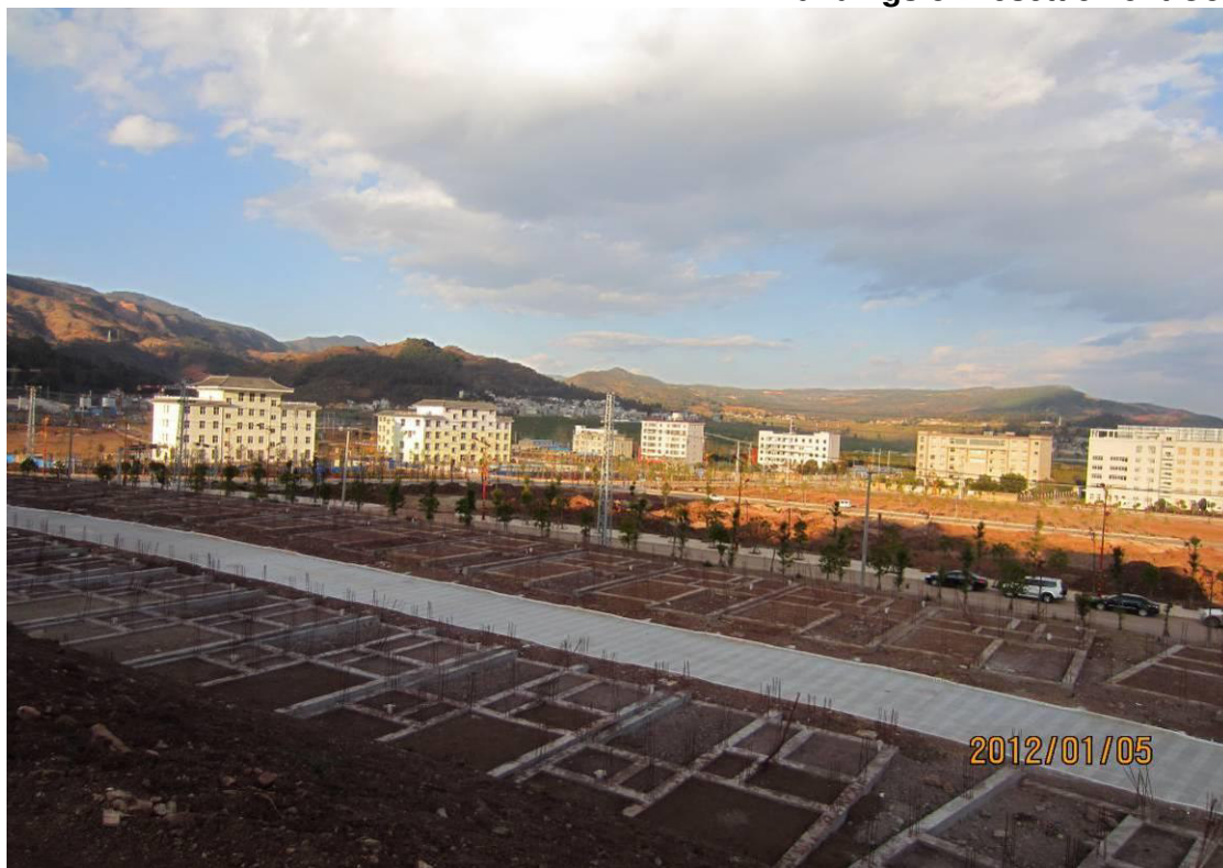
Figure 5-3: Real Photo of Resettlement Site
