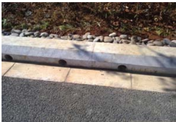
Figure V-3: Curbs with Holes 35
