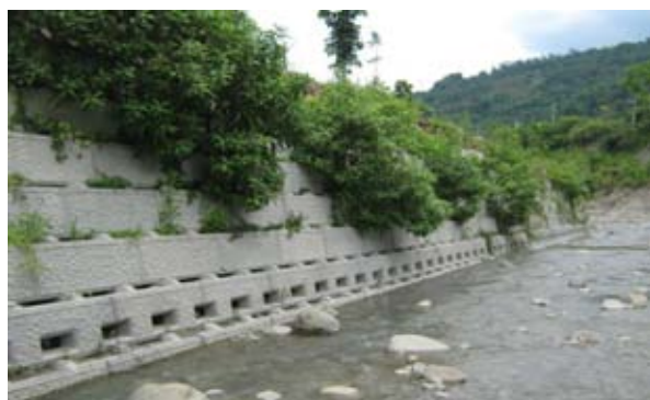
Figure VI-1: Ecological concrete precast block embankment (selected option for Section 3 of Longchuan River, Wuding River)
