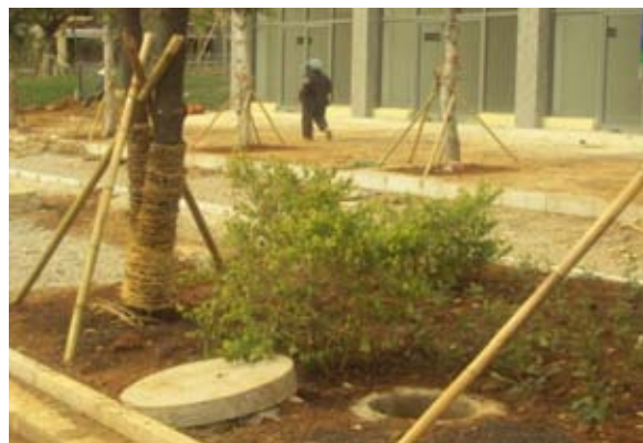
Figure V-4: Rain Water Collecting Wells on Greenbelt
