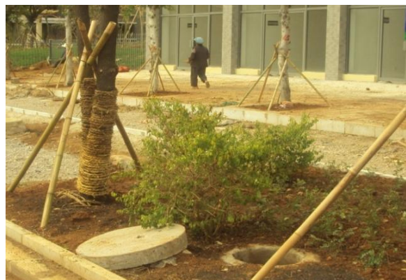
Figure V-4: Rain Water Collecting Wells on Greenbelt
