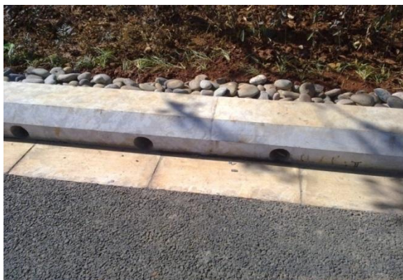
Figure V-3: Curbs with Holes 33
