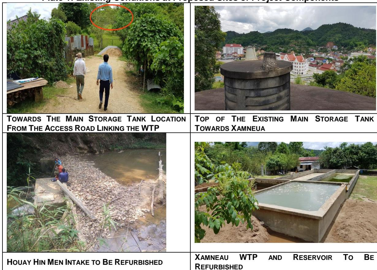
106. It is proposed to rehabilitate and maintain as much of the existing arrangements as possible, but to limit the raw water abstraction from the two houays to about 2,500m<sup>3</sup>/day to enable base environmental flows in the dry season. It is proposed to:
