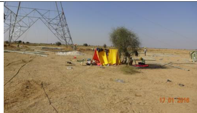
1.6 Temporary camp at tower erection site for tools etc.
