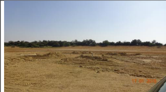
1.9 After construction of foundation of tower foundation before leg erection
