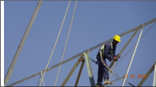
1.7 Use of PPE during tower erection
