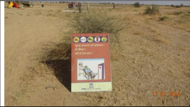
1.8 Display of Safety Boards at construction site.
