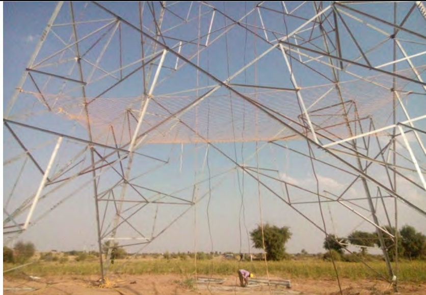
1.7 Usage of Safety Net during erection work.
