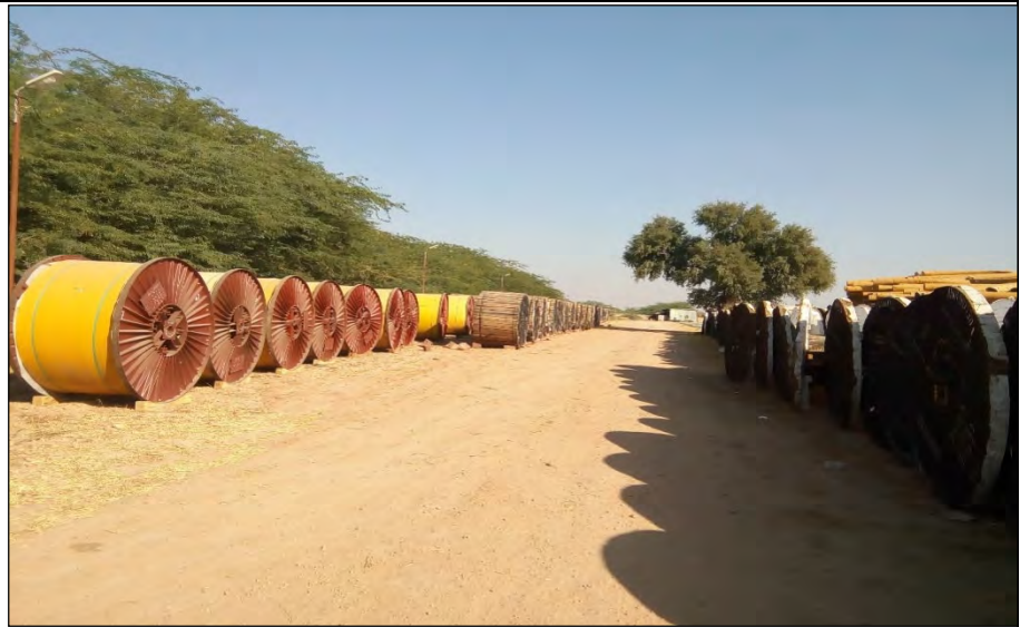
1.6 Storage of ACSR Conductor Drums.
