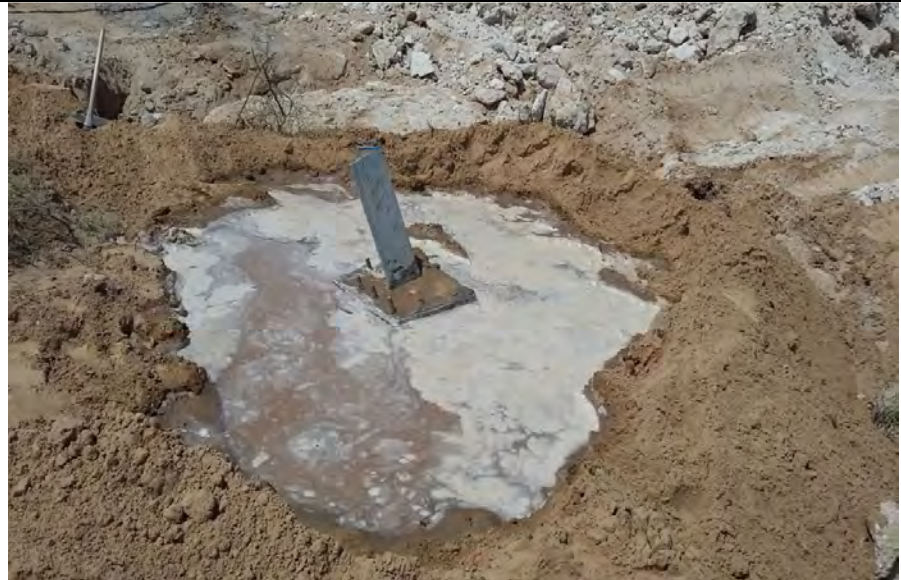
1.8 Usage of adequate water for Foundation curing work
