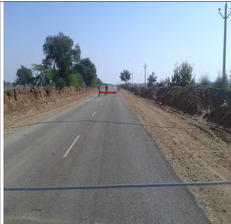
1.7 Safety arrangement during Stringing work.
