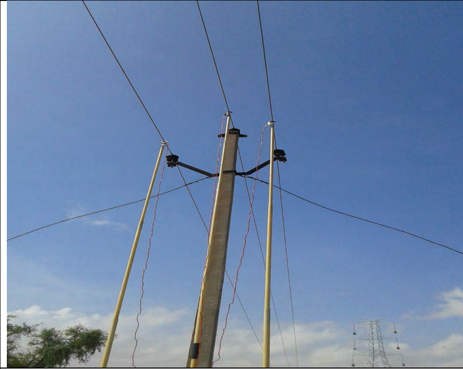
1.5 Use of Discharge Rod During Stringing Work
