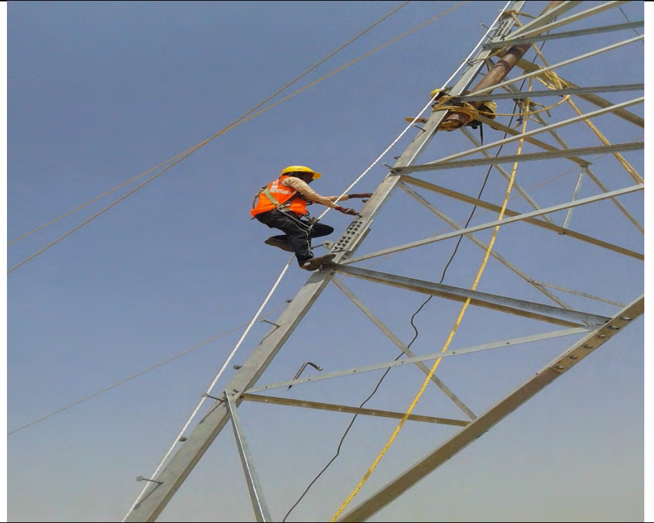
1.4 Implementation of Fall Arrestor during Tower Erection Work
