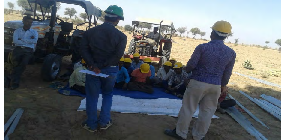
1.1 Safety Tool Box Meeting at site
