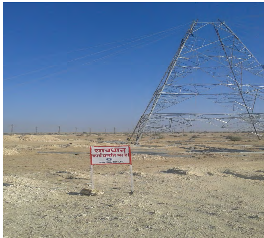
1.8 Safety Banner during Work.
