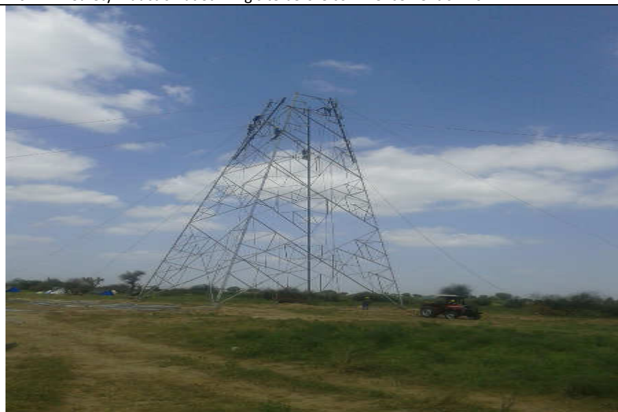
1.8 Tower erection work in progress
