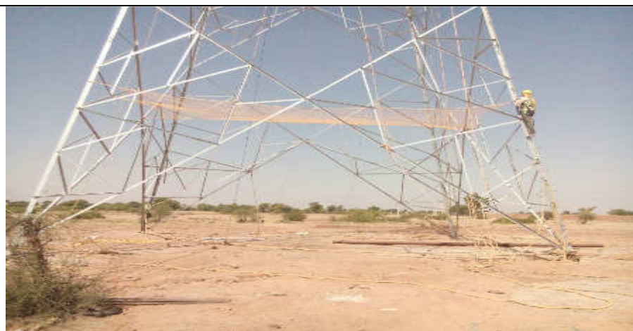
1.2 Usage of Safety Net during the Tower erection work for safety of workmen.
