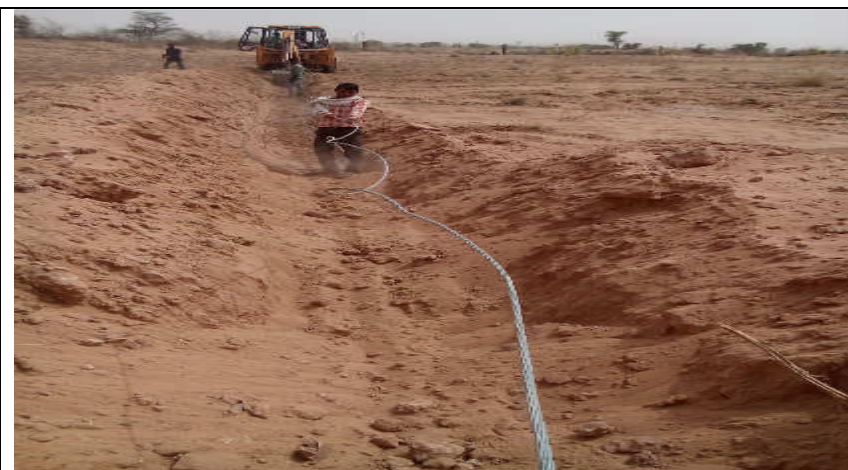
1.1 Laying of Counterpoise Earthing in ground
