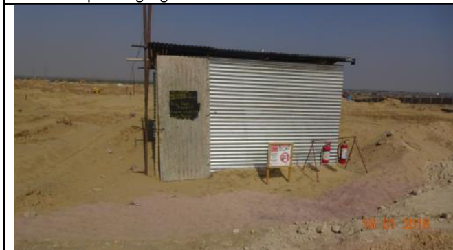
1.13 DG set (Non-silent type enclosure) at site
