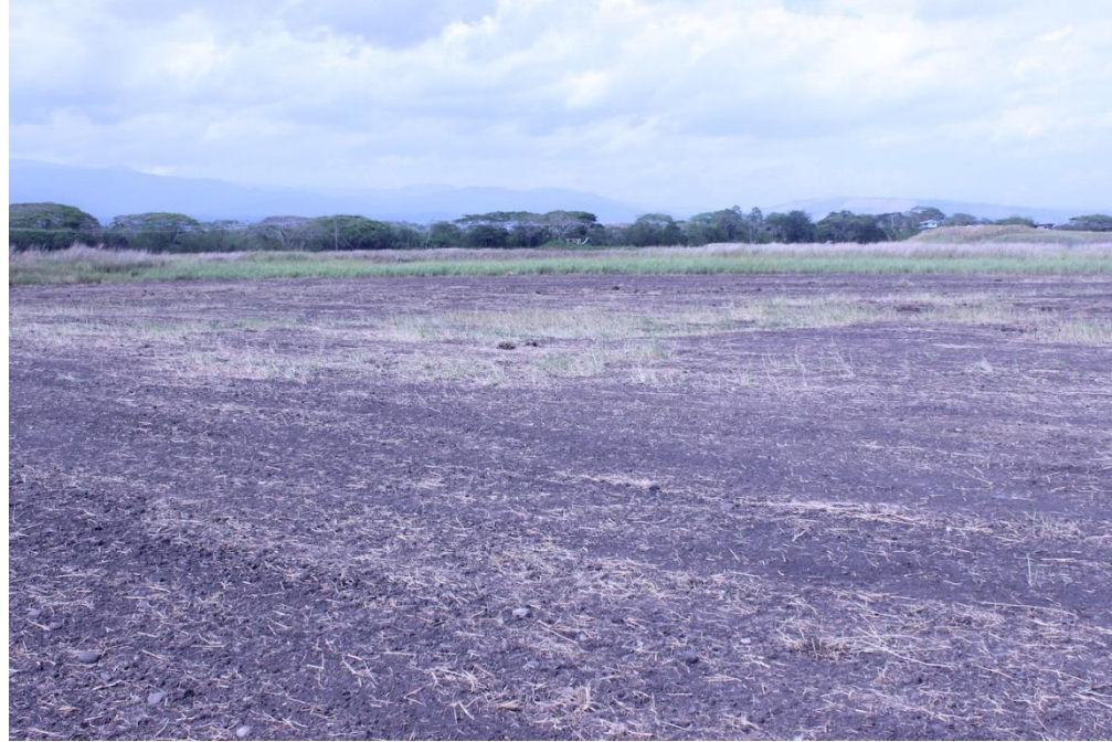
▲ Photo 4 – Pre-construction site clearing and grading in preparation for installation of solar PV arrays and ancillary equipment (2015).
