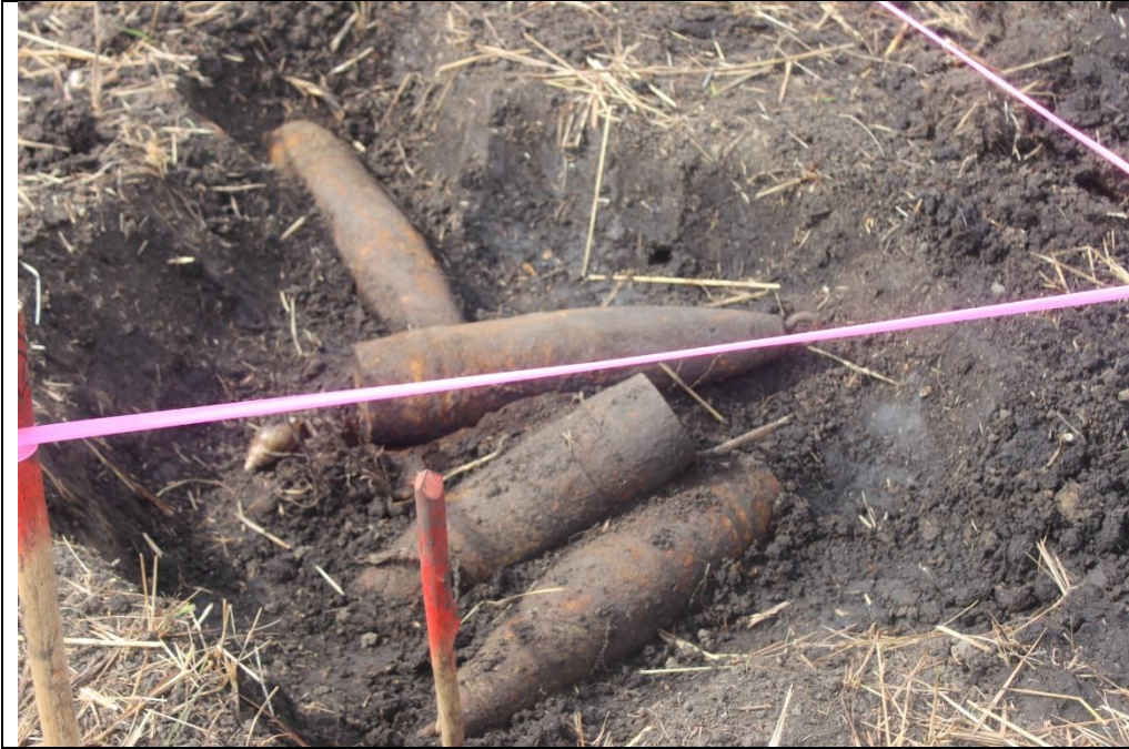
▲ Photo 5 – UXO unearthed at Henderson – Fighter 1 Solar PV site during site UXO survey (2015).
