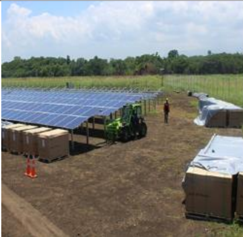
▲ Photo 10 – Solar PV panel installation at Henderson – Fighter 1 solar PV facility (2015).
