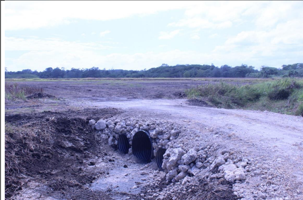
▲ Photo 6 – Culverts installed under access road at entrance to Henderson – Fighter 1 solar PV site on Southwest end of the property (2015).
