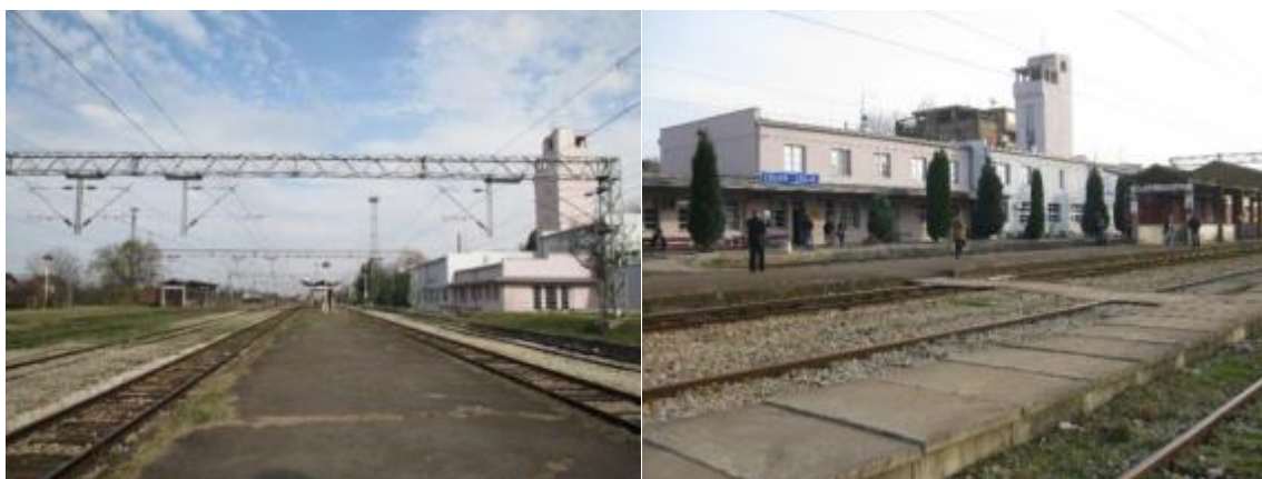
Figure 2 Stalać station – present state
