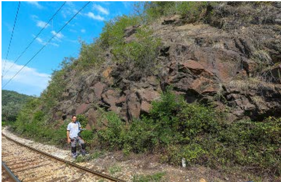
Figure 13 Gneiss rocks in the area of the exit from tunnel 1
