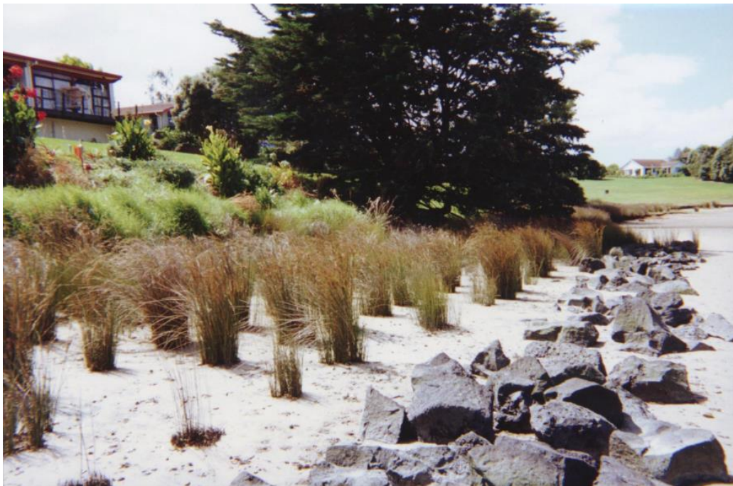
Plate 3.1: Example of riprap boulder placement and planting work
