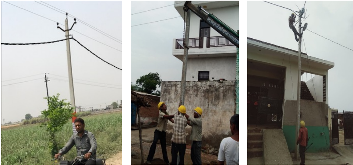
Photo 1: ABC Installation and Stringing Work
