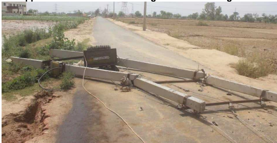
Photo 4: Toppled Distribution Poles in Agra Zone following 2018 Dust Storm
