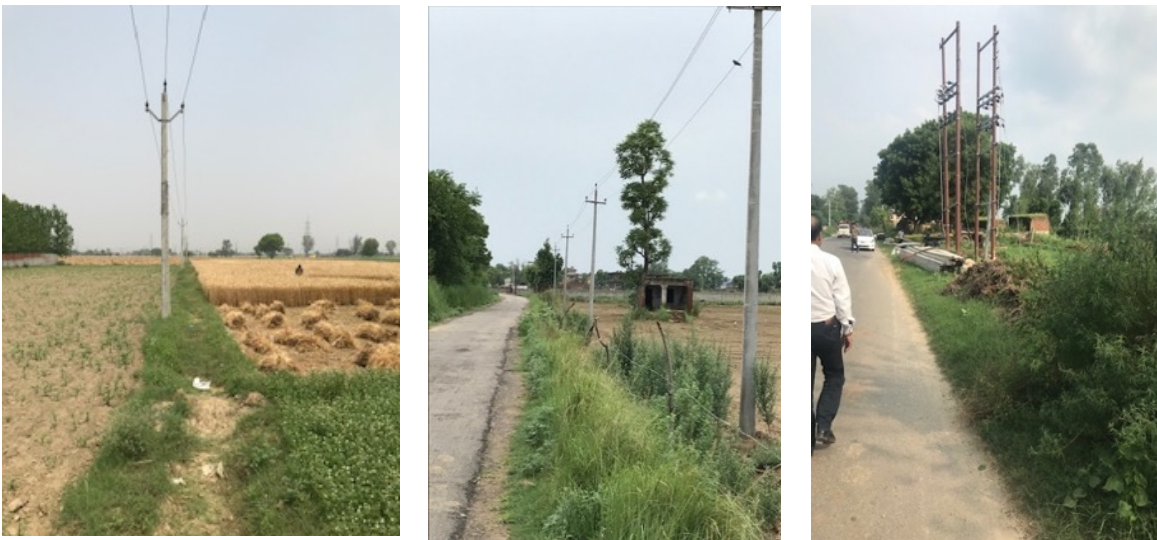
Photo 2: Feeder Separation Works
