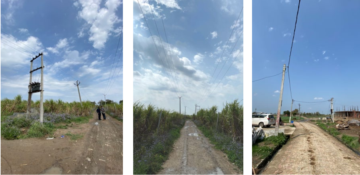
Photo 3: Completed Feeder Separation (left and middle) and ABC (right) Works
