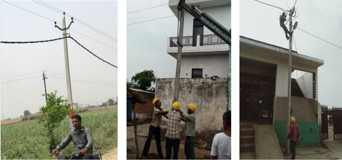
Photo 1: ABC Installation and Stringing Work
