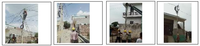
Figure 2: Photographs of ABC Cable replacement work in progress at DVVNL
