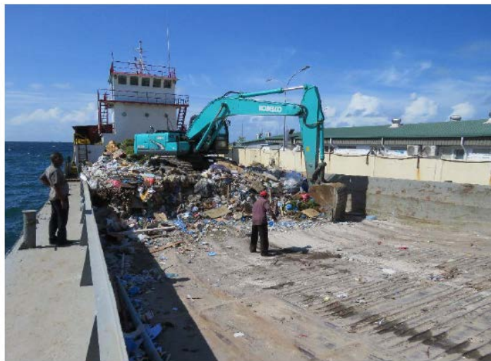
Industrial and C&D Waste Transport at Malé
