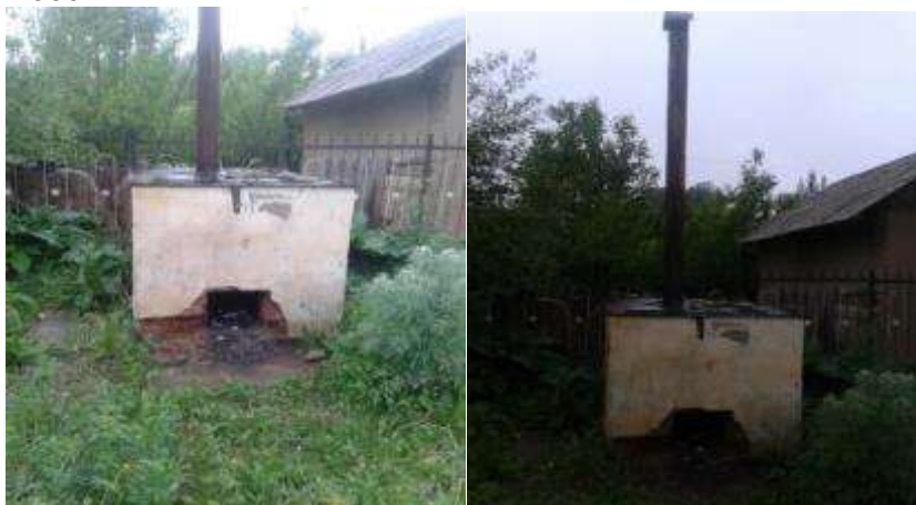
Figure 35: Oven for Burning of Medical Waste at Sh. Shohin DHC
