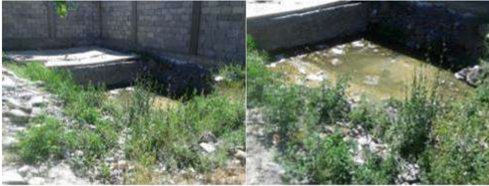
Figure 40: Special Pits for Septic Waste at Aini CDH
