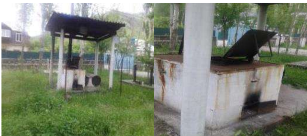
Figure 50: Oven Used for Burning of Medical Waste at Sangvor CDH
