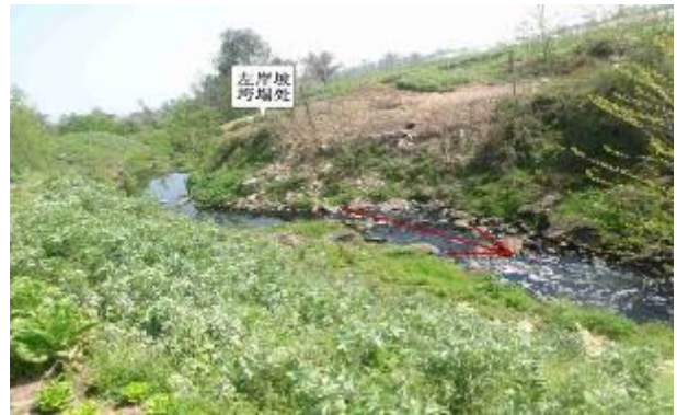
Figure IV-10 Downstream of Baisha River – Bank failure (Liangping)
