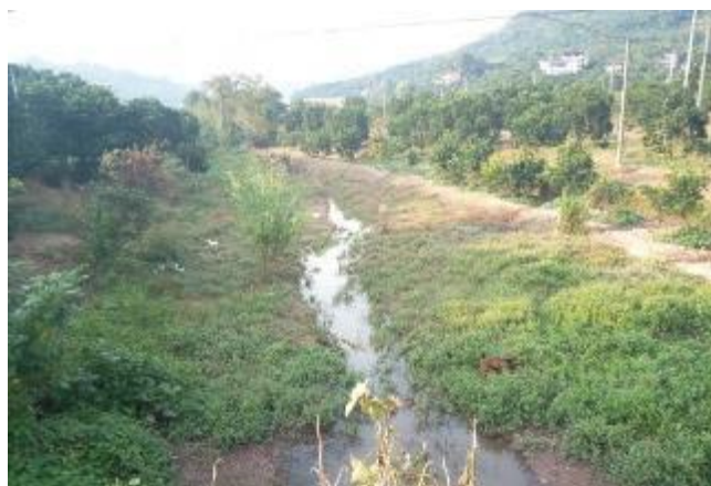
Figure IV-13 Lanjia River – no protection banks (Changshou)
