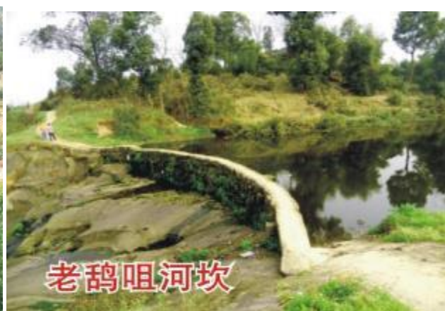
Figure IV-14 Shuanglong River - River weir obstructs flood discharge (Changshou)
