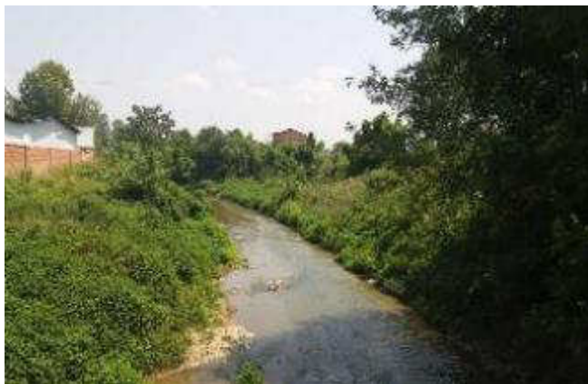
Figure IV-11 Dayu Stream – serious siltation (Dianjiang)
