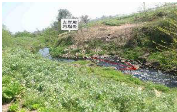
Figure IV-10 Downstream of Baisha River – Bank failure (Liangping)
