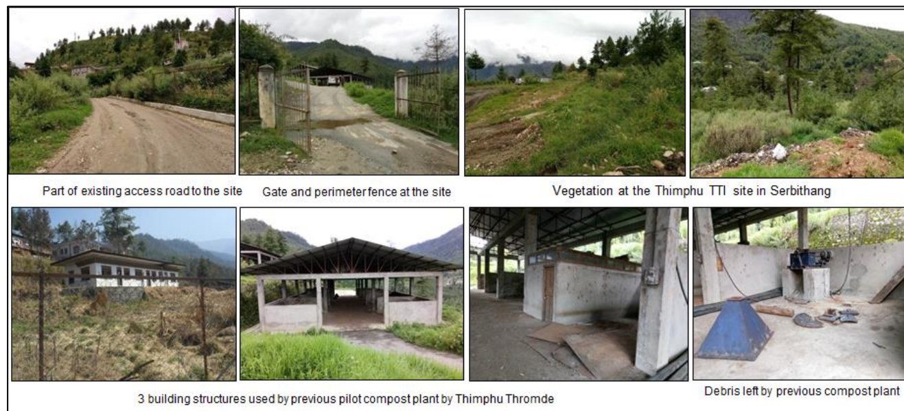
Figure 4.4 Site for the new Thimphu TTI in Serbithang, Thimphu
