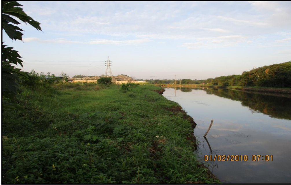
Existing View of the Downstream Garbage Dumping Project
