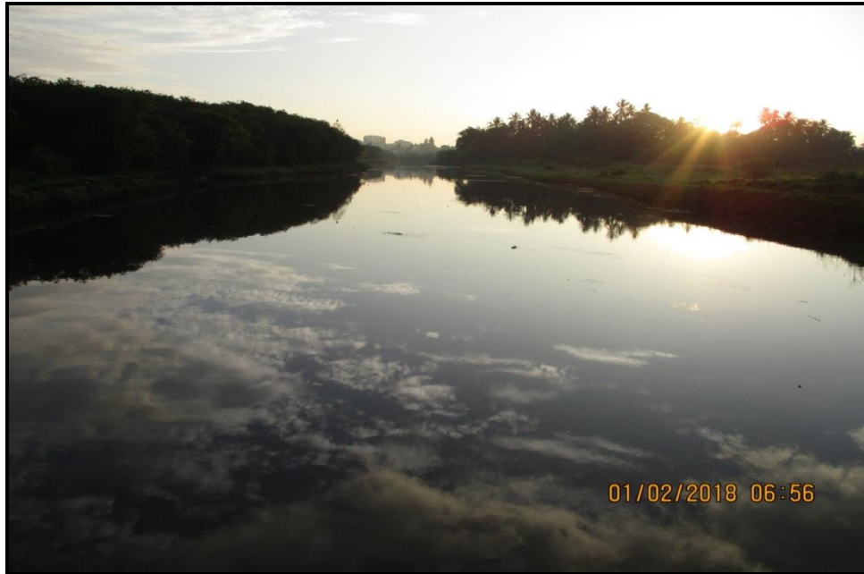
Existing View of the Downstream Main Canal
