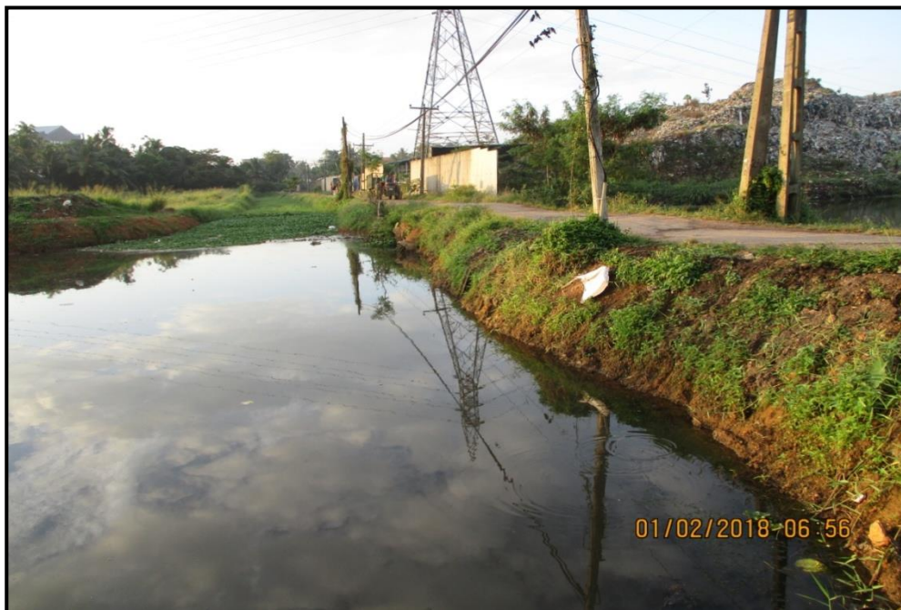
Existing View of the Upstream of the Pipe Culvert Across the Main canal (Opening is not adequate) - Minimum requirement is 30 m span bridge
