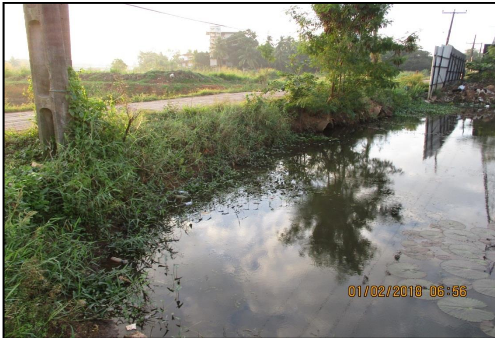
Existing View of the Downstream of the Pipe Culvert Across the Main canal (Opening is not adequate) - 30 m span bridge
