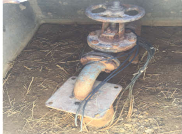
Picture 20: Not operating ground water well
