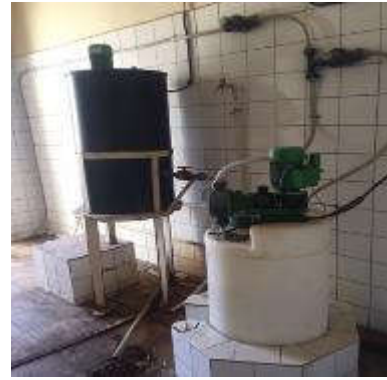
Picture 37: Chlorination facilities on Shortanboy WDC
