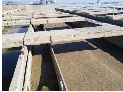
Non-operating longitudinal clarifiers
