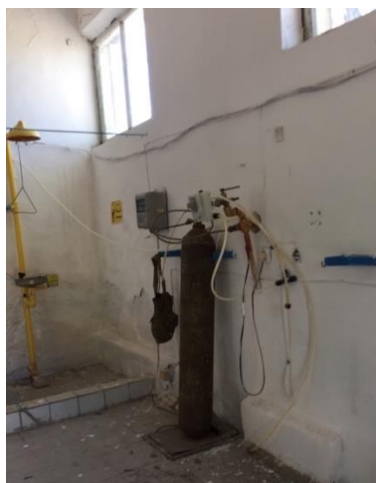
Chlorination facilities at Altinkul WI
