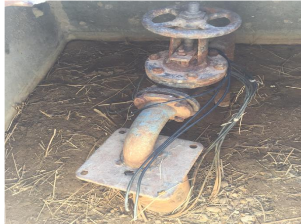
Picture 20: Not operating ground water well
