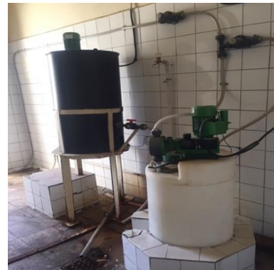
Picture 37: Chlorination facilities on Shortanboy WDC
