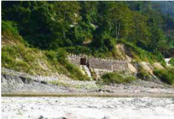
Fig. 1.3 Site photo showing outfall
