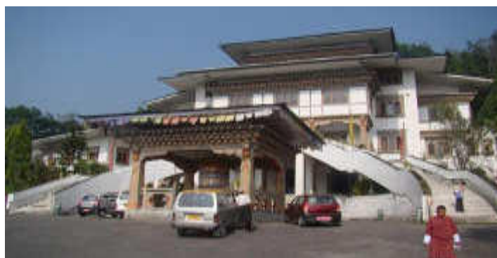
Fig. 2.16 Phuentsholing General Hospital (Source: HCP)
