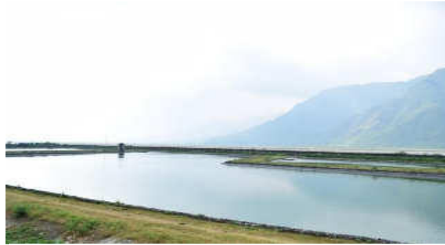
Fig. 2.13 Sewage Treatment Plant (Source: HCP)
