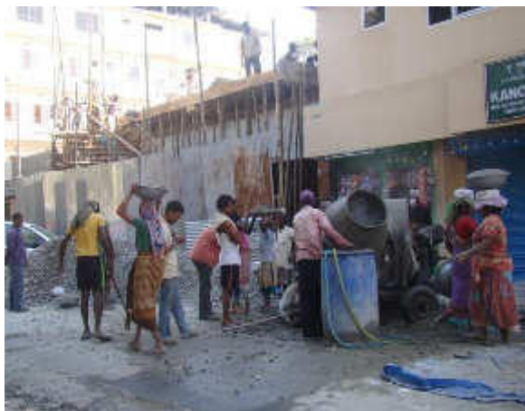
Fig. 2.5 Construction work – Indian labours (Source: HCP)
