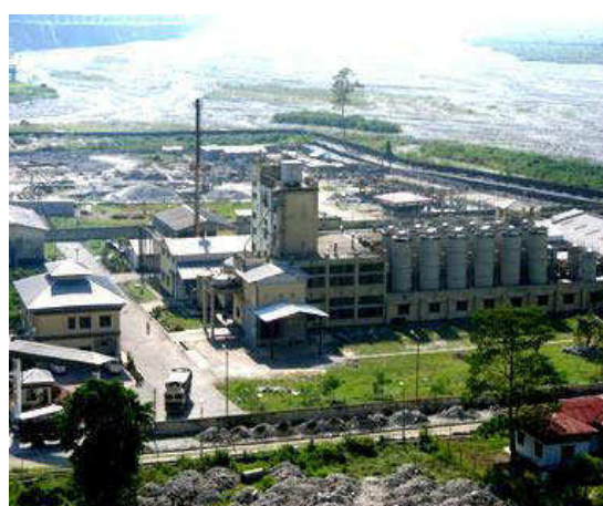
Fig. 2.8 Pasakha Industrial Area – manufacturing industries (Source: tashigroup.bt)
