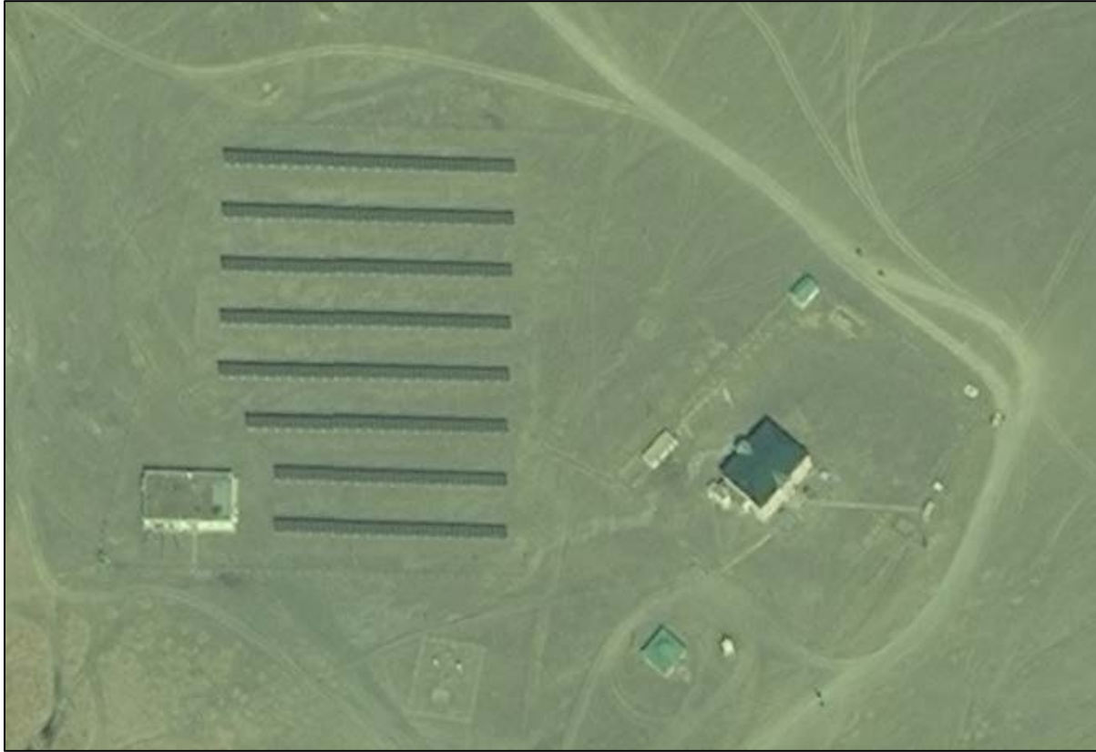
Figure 20: Existing power plant, Altai Soum.
