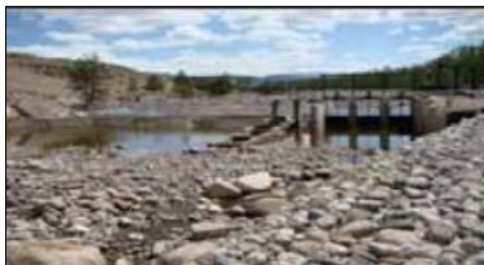
Figure 14: Bogdiin gol run-of-the-river SHPP weir and fish ladder.
