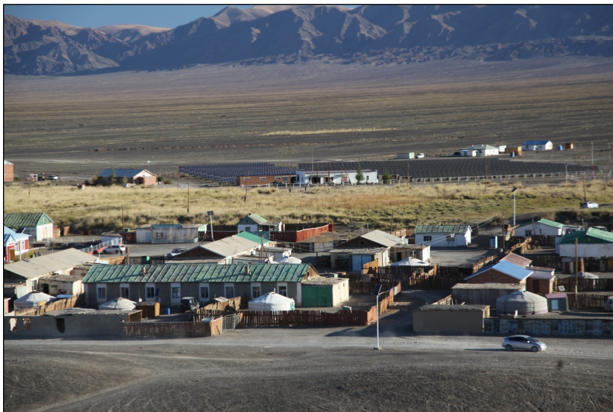
Figure 21: Existing 200 kW PV farm as seen from Altai Soum.
