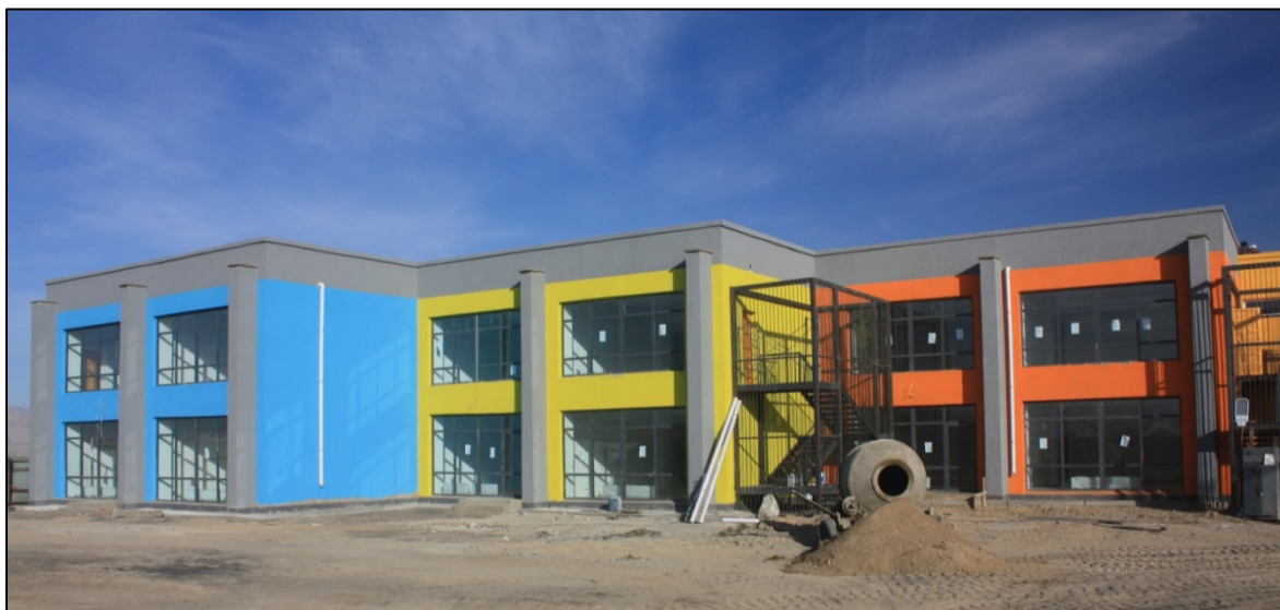
Figure 28: Kindergarten 1 nearing construction completion, October 2017.
