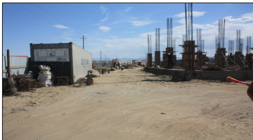
Figure 72: Site conditions at Kindergarten 1, while under construction.
