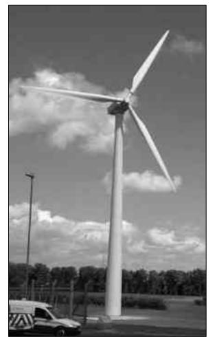
Figure 26: Example of a Wind Technik Nord WTN 250 kW wind turbine.
