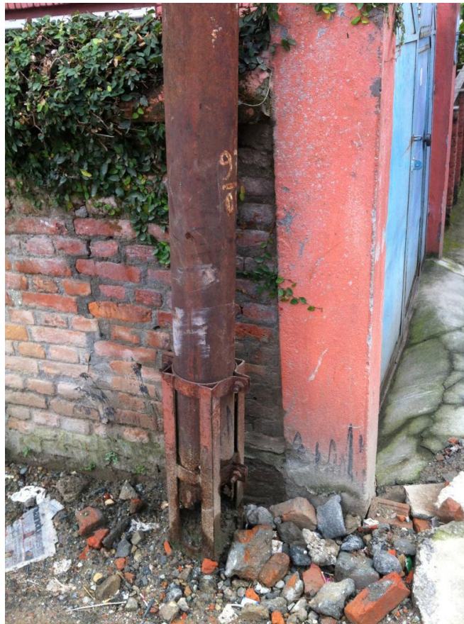
Photo 6: Corroded Poles in Lainchaur Area.
