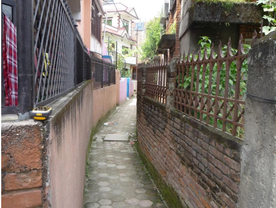
Photo 3: Narrow Residential Road where distribution lines are to be buried
