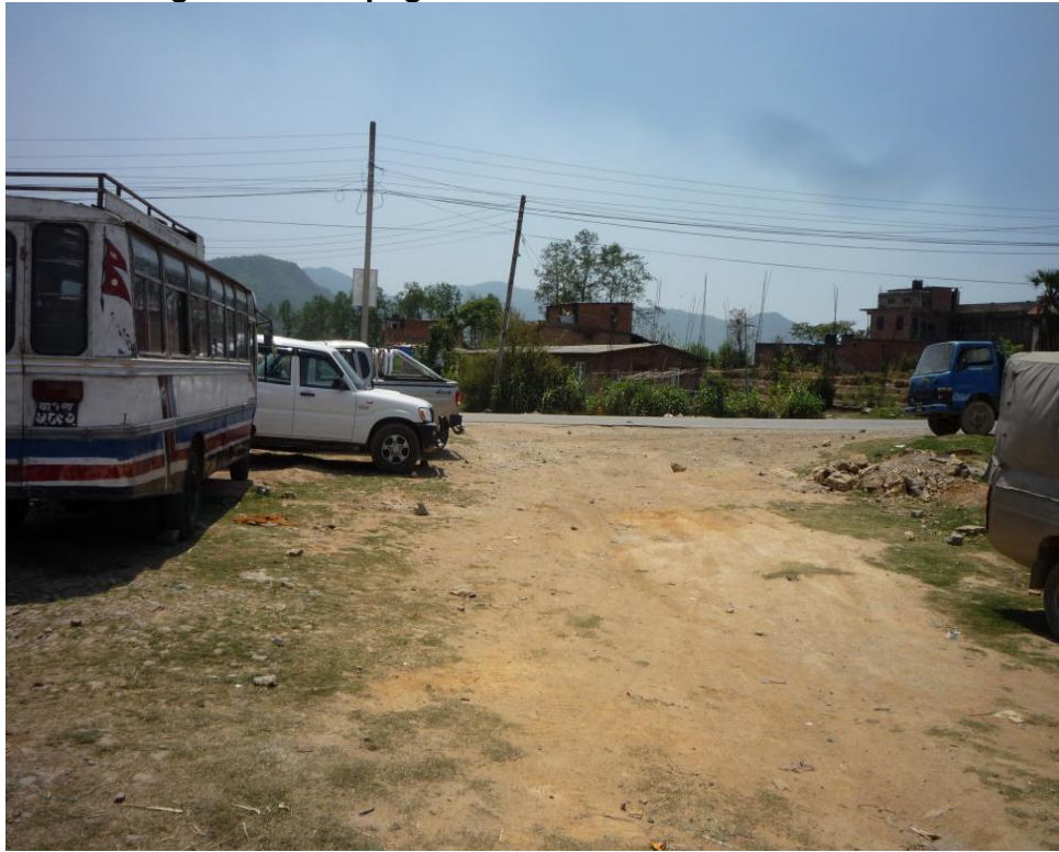
Figure 20: Chapagaun Substation Site Access Road
