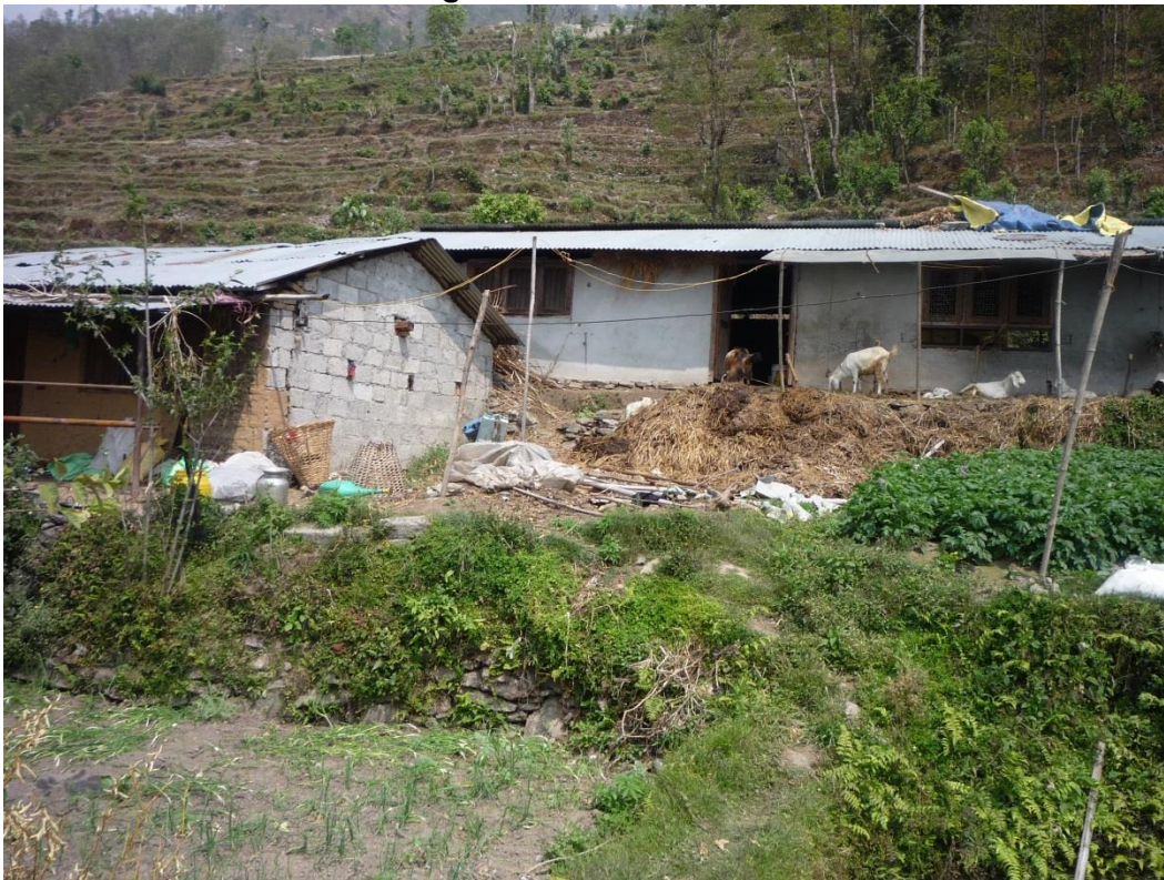
Photo 8: Existing Structures in Barhabise Substation Site.
