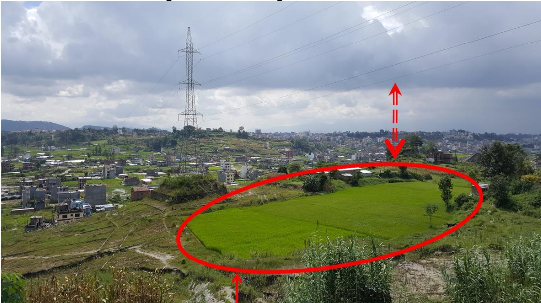
Figure 16: Phutung Substation Site
