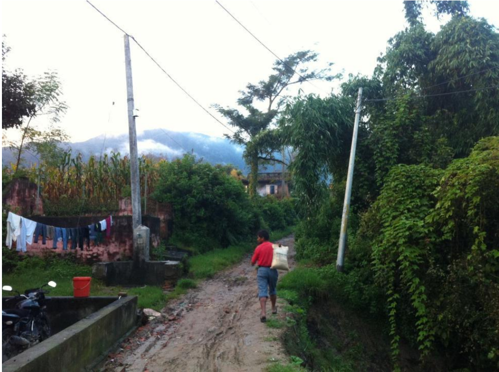
Utility Poles in Unstable Areas - Dharmasthali
