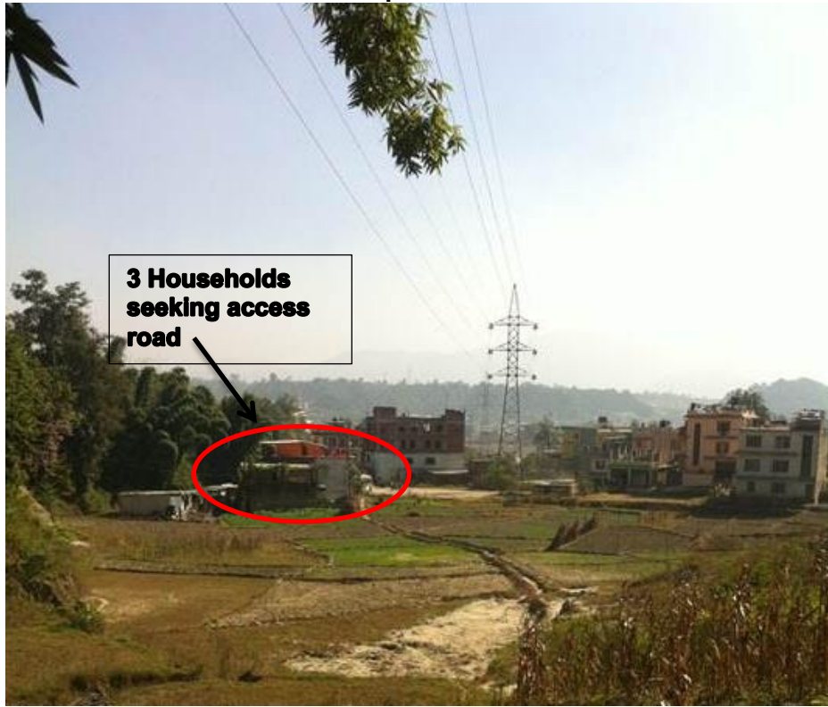
Photo 1: Moolpani Substation Site
