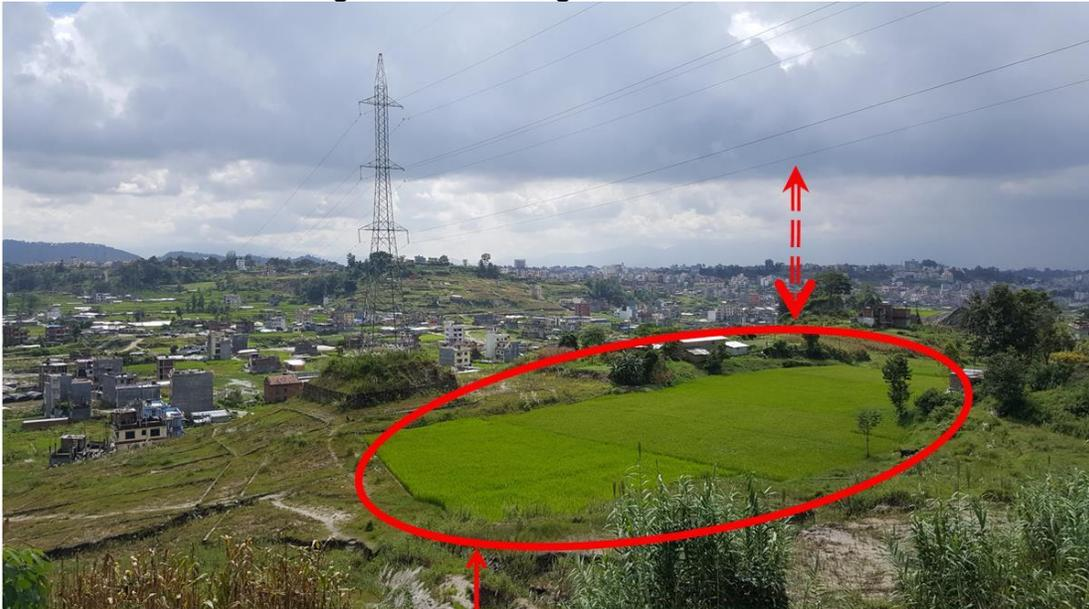
The substation will connect to existing overhead 132 kV lines with a vertical loop-in / loop-out design, minimizing the overall footprint. An access road of less than 100 meters will be required.
