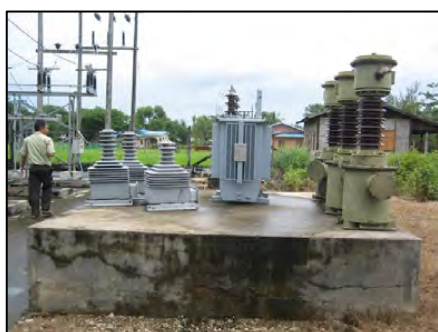
The existing transformer and SF 6 circuit breakers at the substation.
