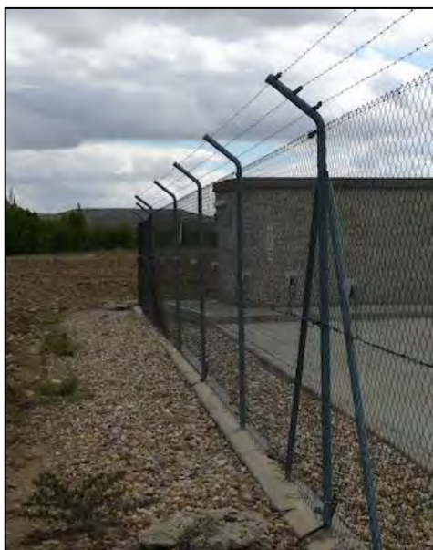
Example of galvanized mesh wire with outgoing anti-climbing section
