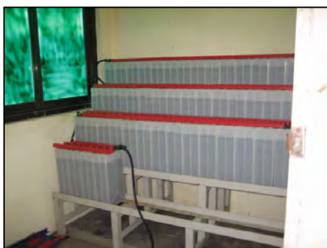
Battery charging area inside the substation building.
