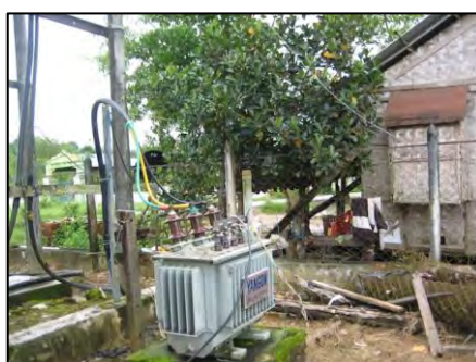
There is very limited space and protection between the adjacent house and the transformer with open wires.
