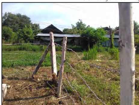
Only barbed wire is used as fence of the substation.
