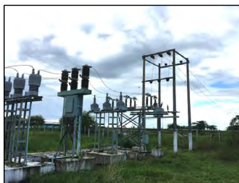
The switchyard with SF6 circuit breakers.
