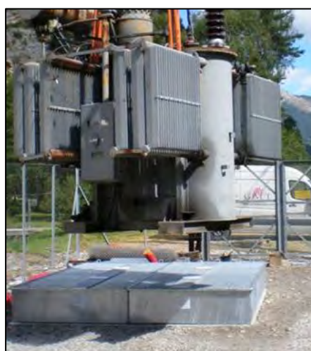
Example of oil pit for large transformer
