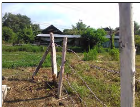
Barbed wire fence in existing Thegon substation which will not prevent people and animals from entering the substation compound.
