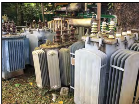
Damaged transformers outside the warehouse building.
