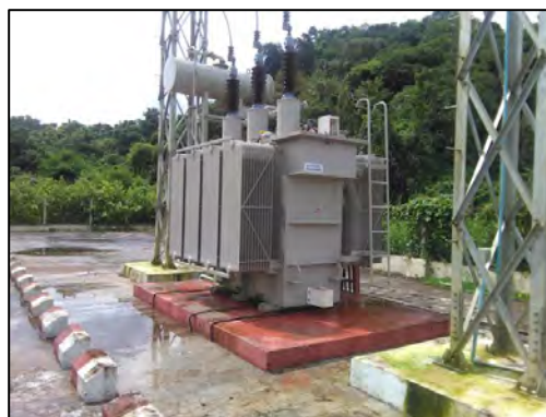
A 66/11 kV transformter at Nga Yoke Kaung installed in 2015 but no oil containment. The transformers are standing on concrete foundation.
