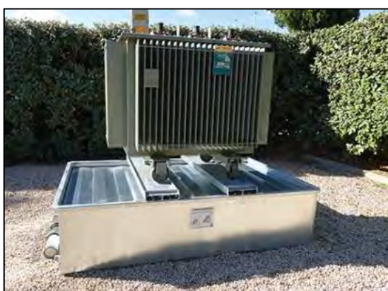
Example of oil pit with filter system for small transformer
