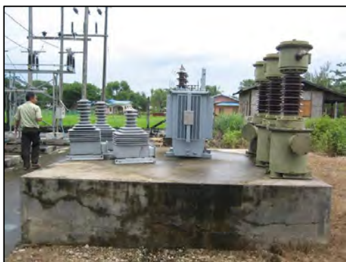
The transformer platform at Oktwin substation but without oil pit.
