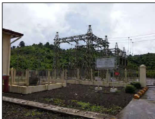
Fence at Nga Yoke Kaung substation which was installed in 2015. The fence is quite sturdy and includes a concrete foundation to prevent animals from entering under the fence. However, the fence is not high enough and one can easily go over it.
