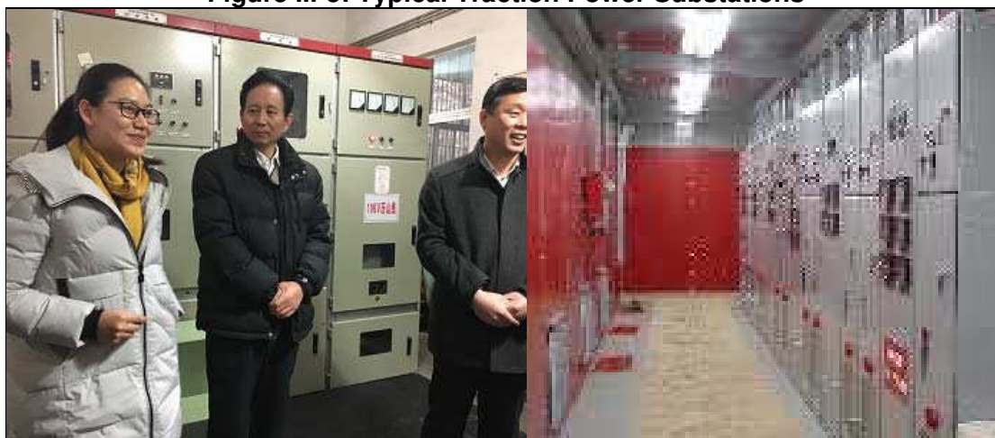
Figure III-5: Typical Traction Power Substations
