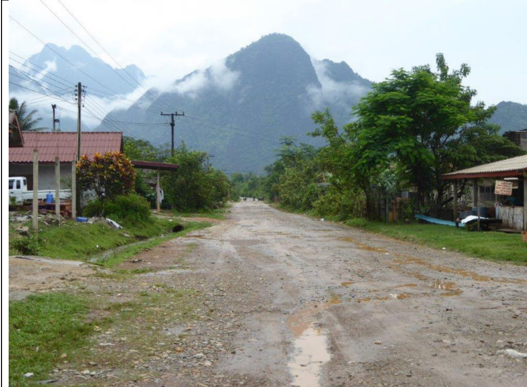
Figure 24c: Example section of western link road to be upgraded.
