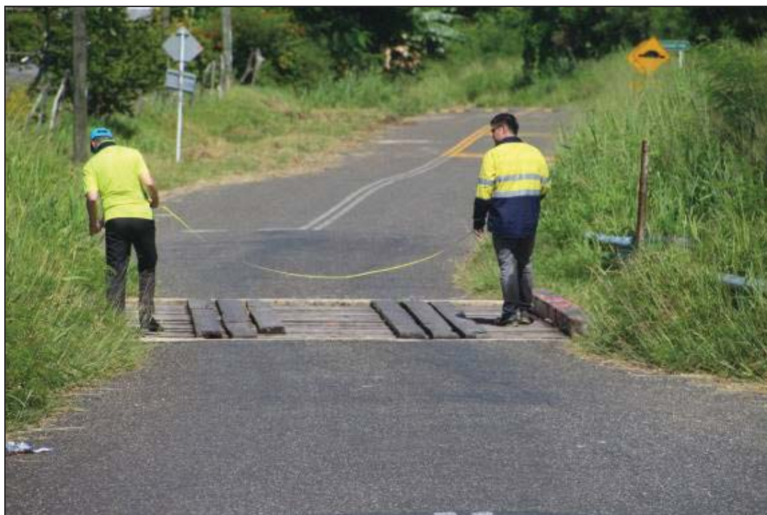
Figure 3-2 Engineering inspections at Ulei Bridge
