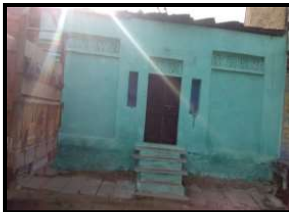
Residential Encroacher - km24.355 of SH-74 (RHS) - Mr. Ramrup Kumhar - House
