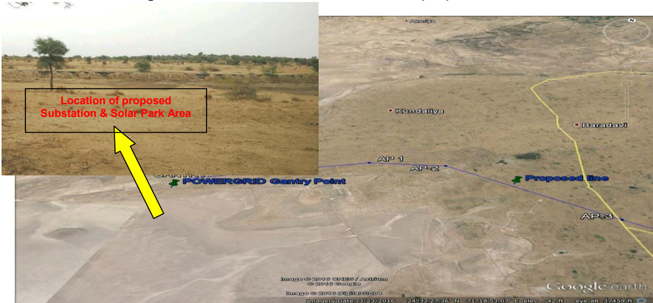
Figure 3.3: PG Gantry location at proposed 400/220/kV Radhanesda (GETCO) Substation
