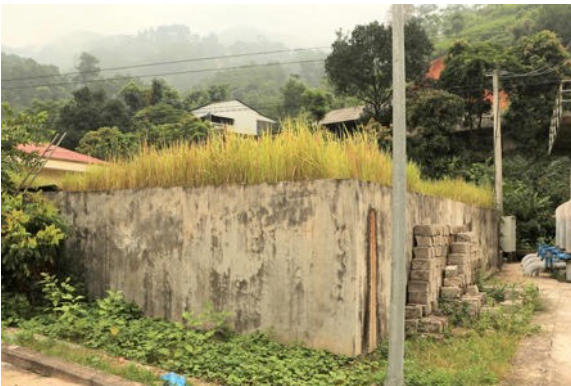
Grass grow on top of sludge tank as a natural cooling system
