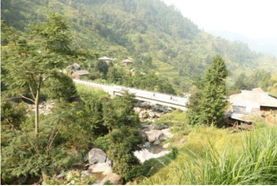
Overview of water intake area (Pin Ho bridge)
