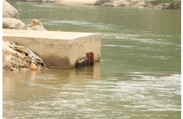
Water intake of the existing water supply in Chay River
