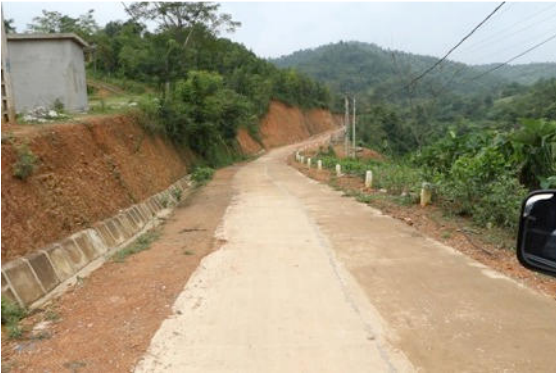
Good road section near Quy Hoa CPC
