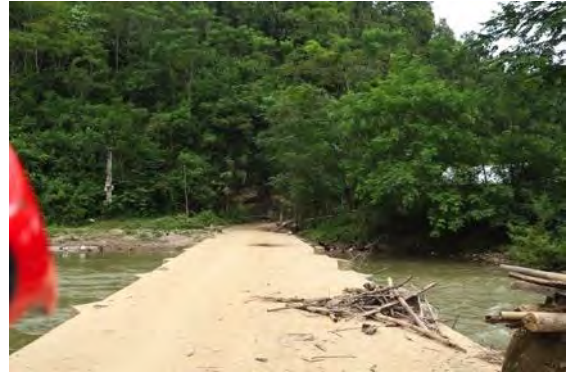
Khuoi Man concrete causeway Km22+230
