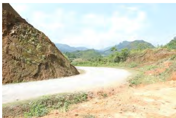
Current road condition at the proposed WTP
