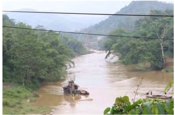
View from the road to Bac Giang River and Bac Giang 1 Hydro Power Plant
