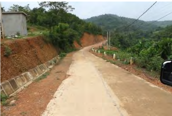
Good road section near Quy Hoa CPC
