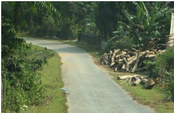
Road section in Dong Tam commune
