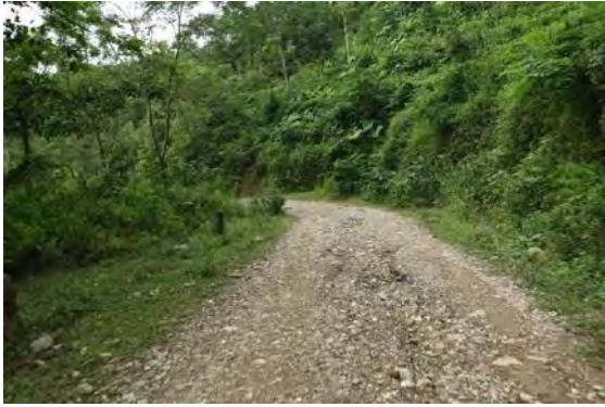
Down grade road section in Bang Thanh
