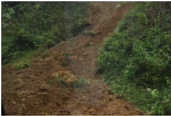
Landslide near the road in Quang Trung commune
