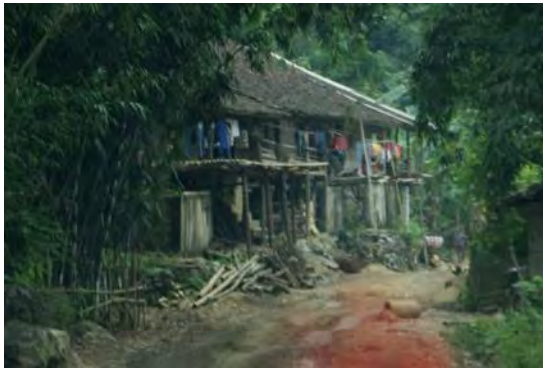
Narrow road section through Ban Ngan village
