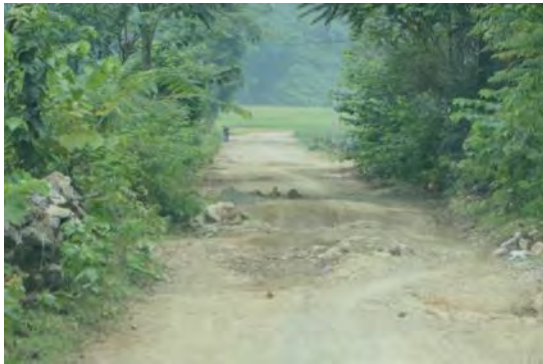
Road section in Xuan Noi commune
