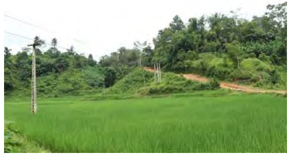
Road section in Quy Hoa commune with large rice field and electric line 0.4kV
