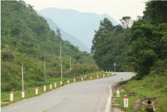
PR203 the main road through subproject area of
