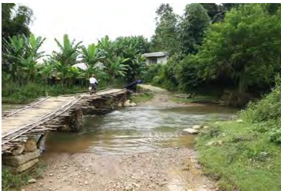
Intersection with Nang River at Km22+650
