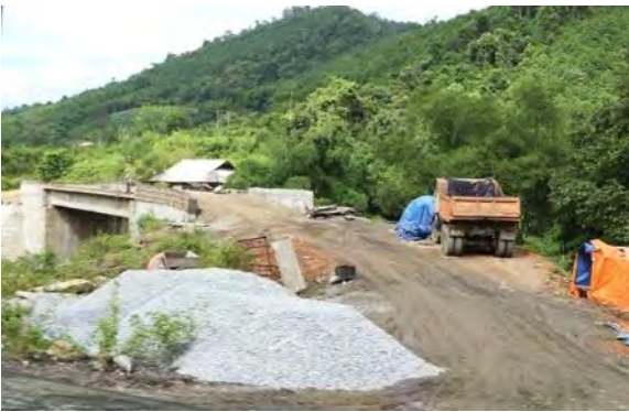
Under construction bridge in Na Lay village
