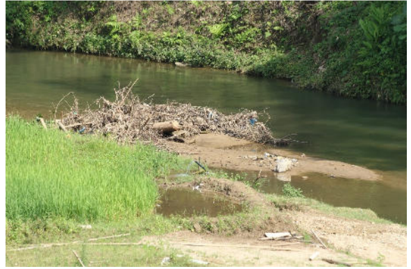
Waste accumulated near Vang My Weir
