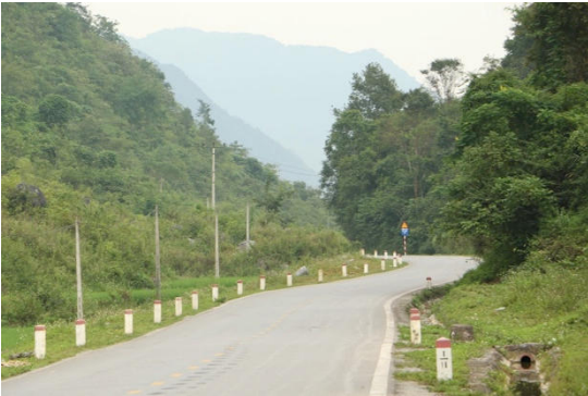
PR203 the main road through subproject area
