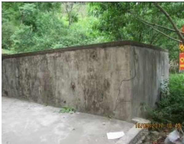
Water tank in Nam Dan commune which made of brick and concrete is cracked
