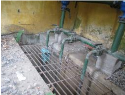
Submerged pumps have been installed but cannot operate because of without electric
