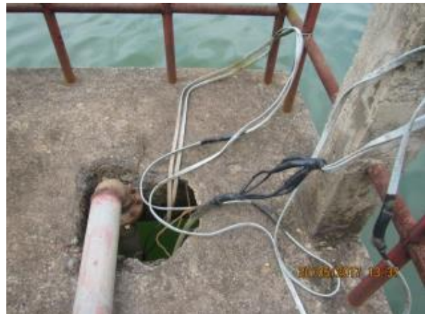
Pump in Thai Binh water source need to be raised capacity
