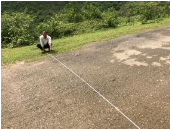
The Ending Point Km4+600 between Xuan Duong - Thien Long
