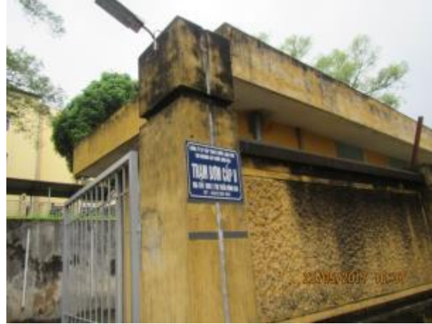
Expanding the current secondary water pump is difficult because of limitation of land area
