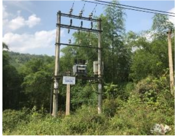
Electric Station at Km0
