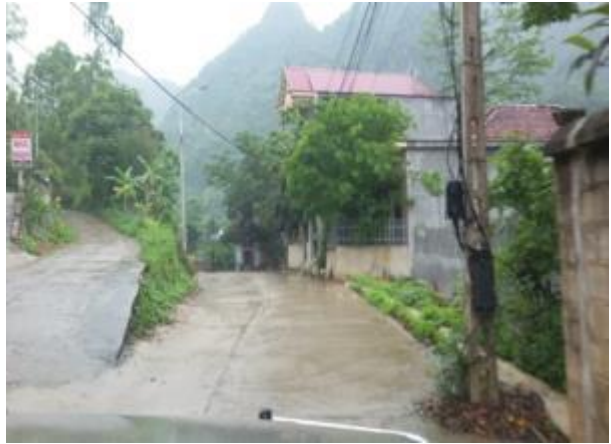
Km0+400 (Cement concrete pavement)
