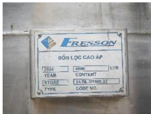
High pressure infiltration tank with capacity 4,500 litter, installed in 2004
