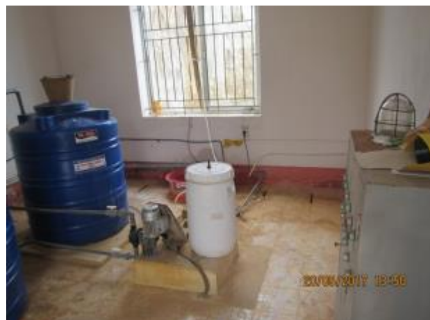
Chemical room in water treatment plant. Chlorine is pumped direct to water tank
