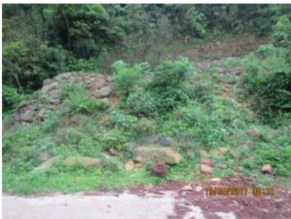
Location for construction of weir in Mau Son area. inflow water data is unavailable
