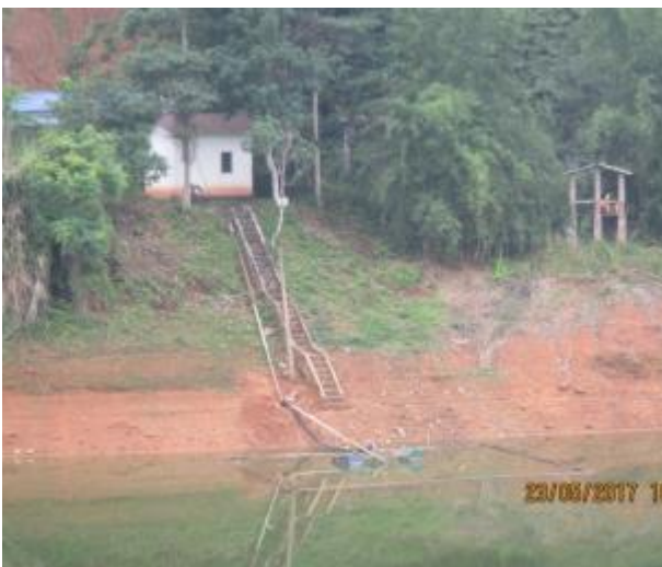
Existing water supply primary pump system for To Hieu commune
