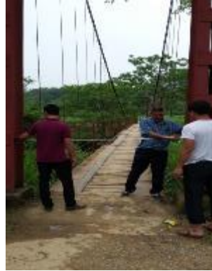
Bac Son suspension bridge over Na Ri river
