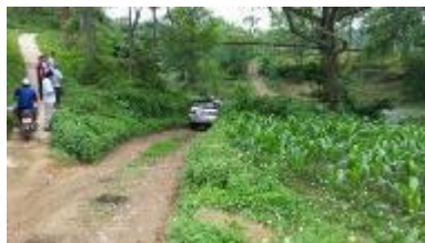
Causeway under Bac Son suspension bridge over Na Ri river
