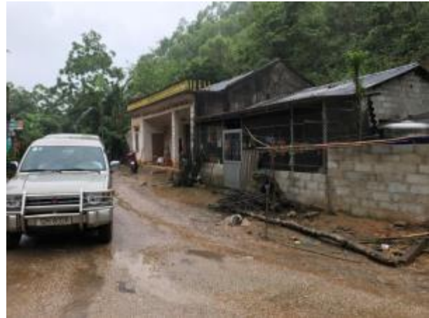
End point Km9+728
