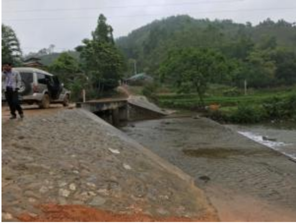
Na Tau Bridge Km4+286
