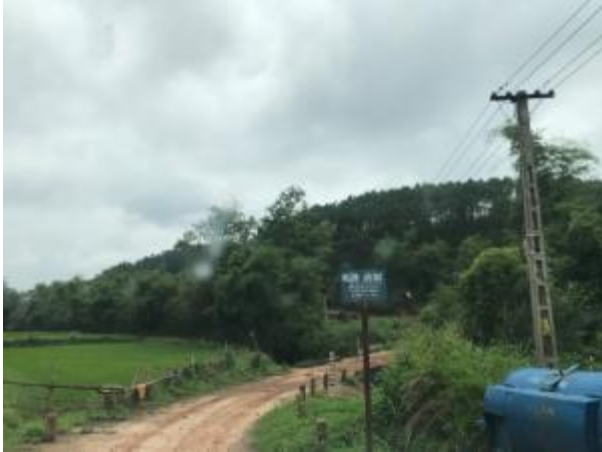
Km16+230 (Bridge Ban Moi) L=5m
