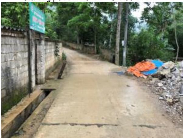
Km0+800 (end section of cement concrete)
