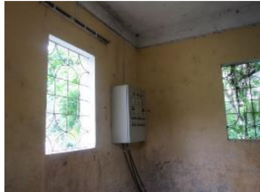
Control box inside pump station does not connect to main electric cable because of transformer was not being installed
