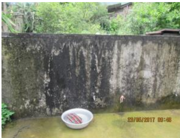
Main brick water tank in Tan Van to store water from gulch without treatment
