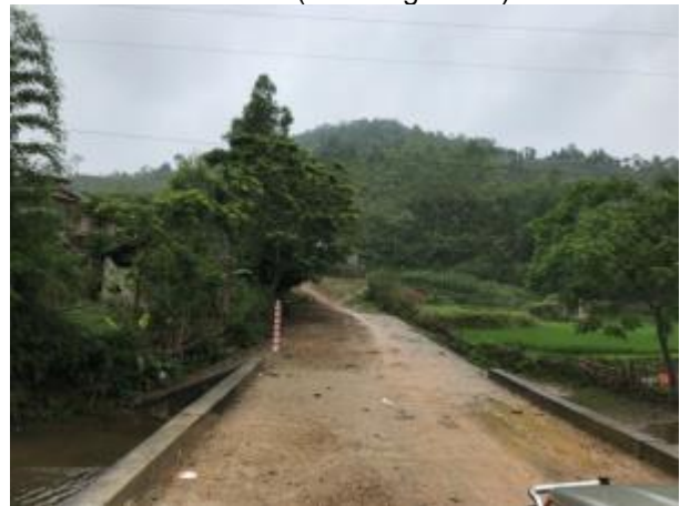
Bridge 4+286: Na Tu Bridge
