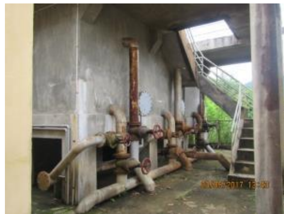
Water treatment plant in Thai Binh town is old and small capacity
