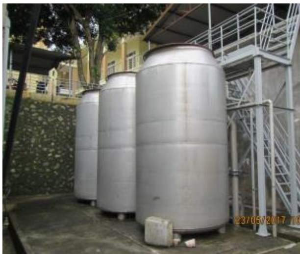
Current water treatment plant for To Hieu commune only but its capacity cannot be extended for other water demand
