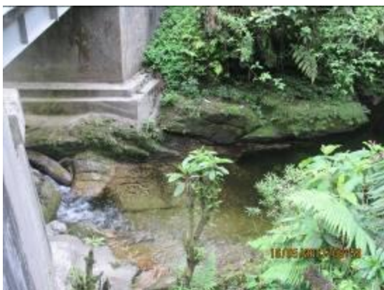
At present time, water quality is reasonable but in rainy season, solid particle and TSS in water increase
