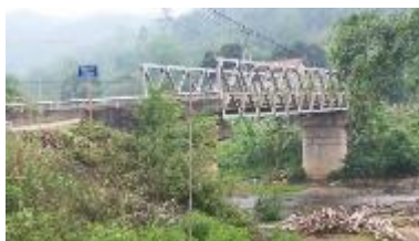
Quang Phong bridge L=58m, and Wdt=4m
