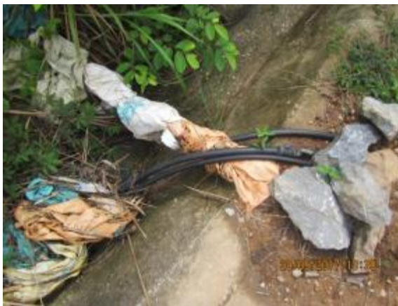
Various water extract pipe erected by local people when water treatment plant was not working
