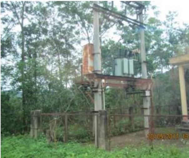
Existing transformer in Thai Binh plant needs to be upgraded
