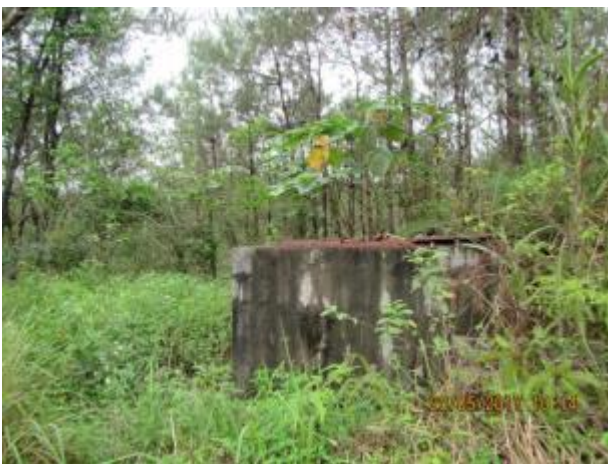
Existing water tank in Khe Bo village is empty
