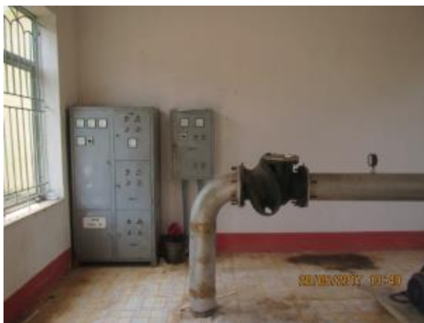
Electric control box in Thai Binh water treatment plant which is using old technology
