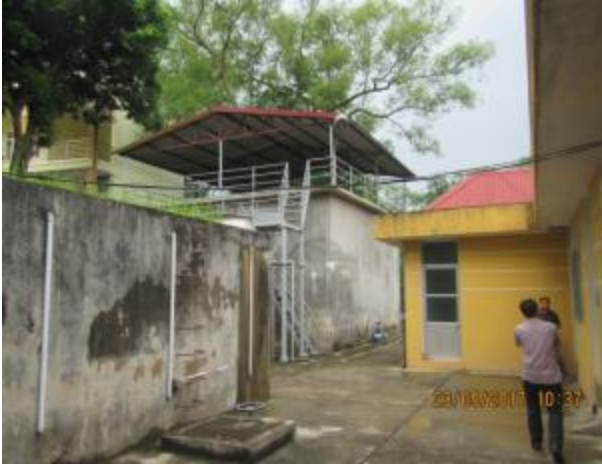
Expanding the current water treatment plant is difficult because of limitation of land area
