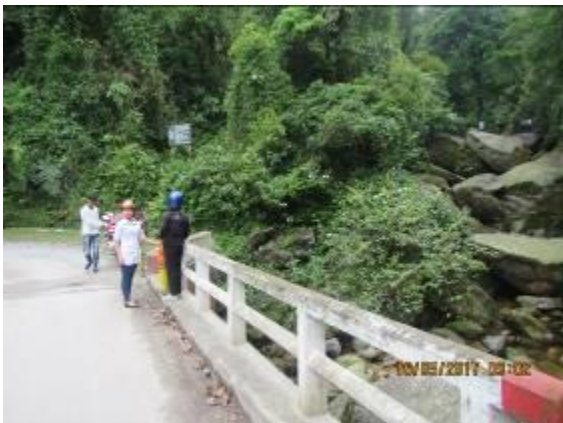
Bridge in Nam Dan stream with high clearance due to peak water flow in flood season.
