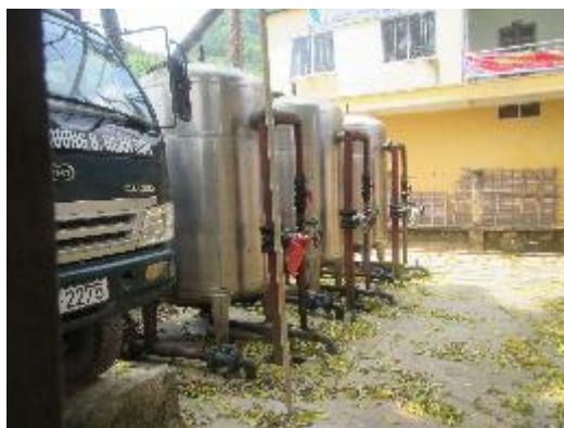
Current 03 infiltration water treatment tanks in Van Tung water treatment plant
