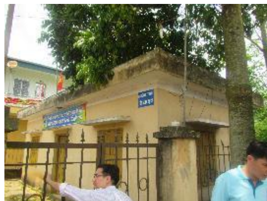
Water treatment plant in Van Tung
