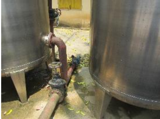
Water treatment equipment is downgraded
