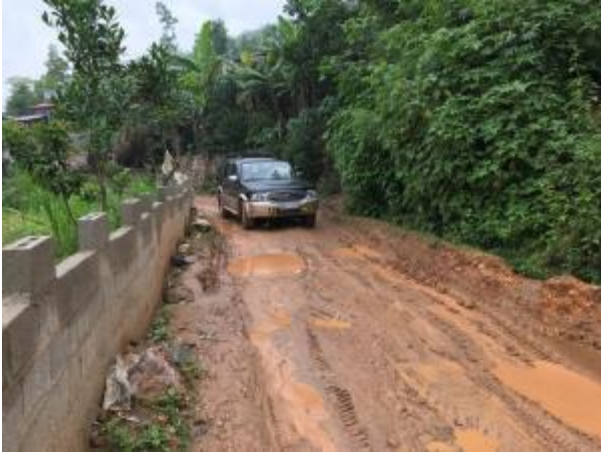
Km2+400 (New alignment)
