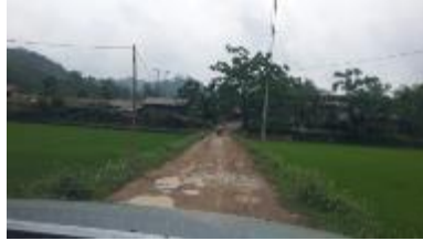
Earth road with lots of potholes and rice field along the road
