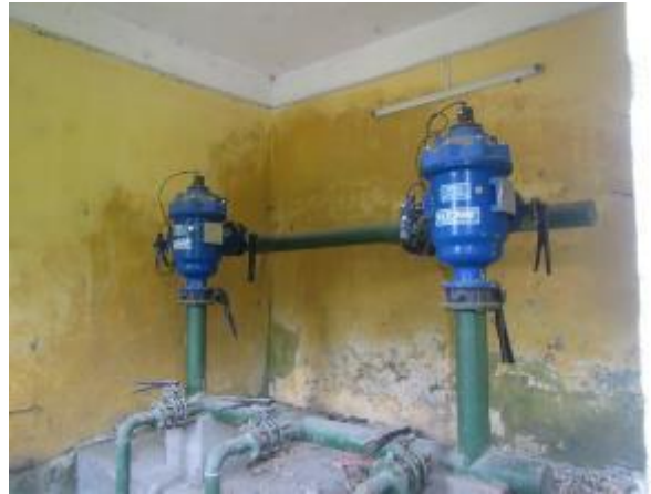
Water treatment equipment constructed but not used
