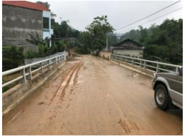
Bridge Na Phai Km0+269
