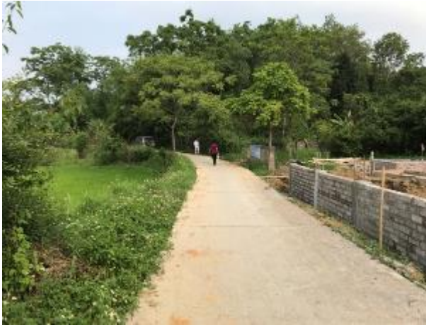
Starting point Connection with NR3B
