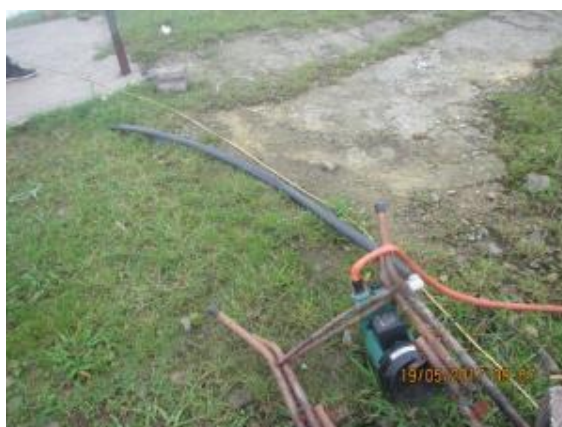
Individual electric water pump. Water is extracting from intermediate pond below. Pond was constructed by French in the past
