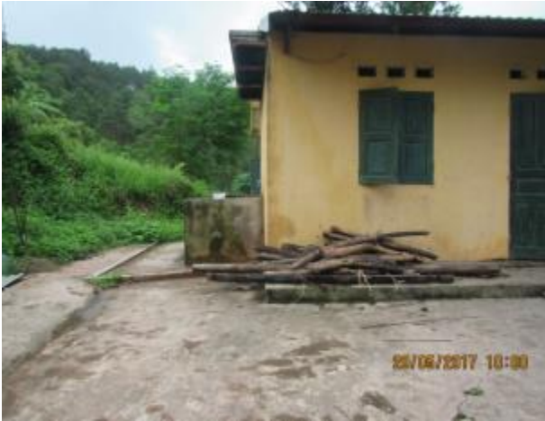
Water tank in Dong Khoang village, which is made of brick and concrete. Water is taken from Dong Khoang stream without treatment facility
