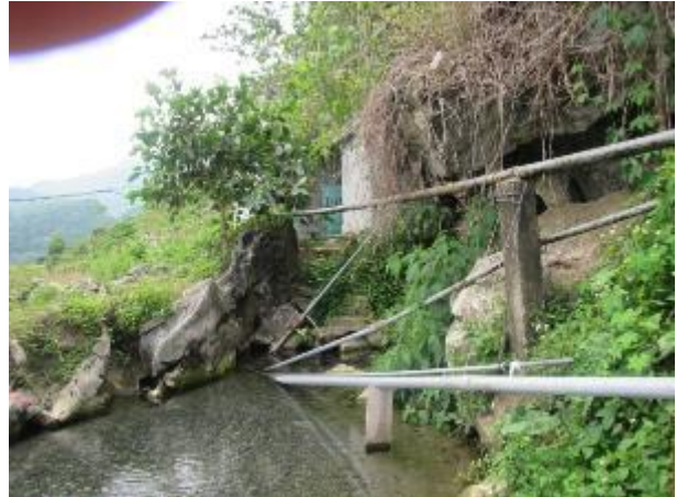
Various extract pipe to collect water from natural water source for Pac Miao School, Police Station, Military office and local people
