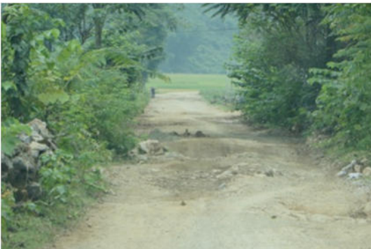
Road section in Xuan Noi commune
