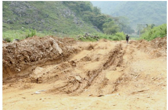
Bad road surface section in Lang Yen commune
