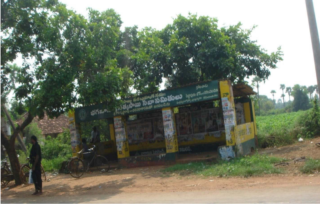
CPRs Bus-Stand At Kotapadu Village Chainage 17+370
