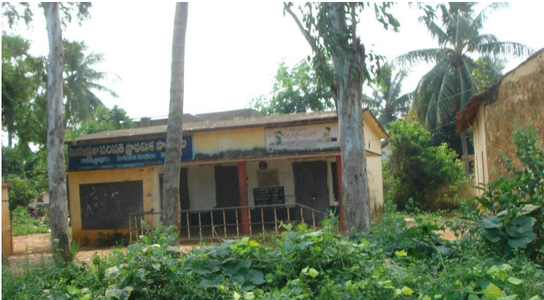
CPRs MPPS At Kotapadu Village Chainage 17+280
