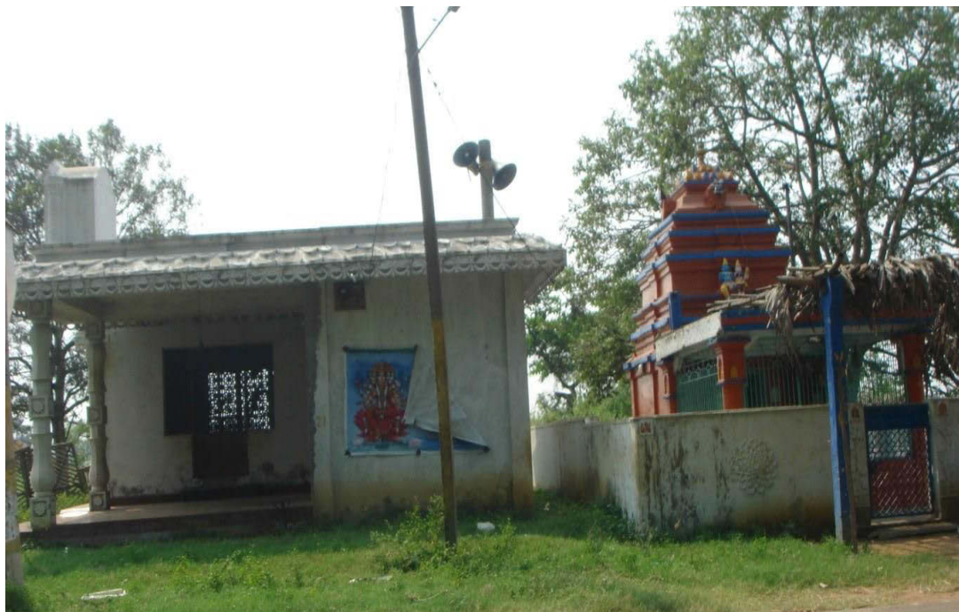
CPRs Vedhamatha Temple & Haman Temple At Vadiseleru Village Chainage 26+500
