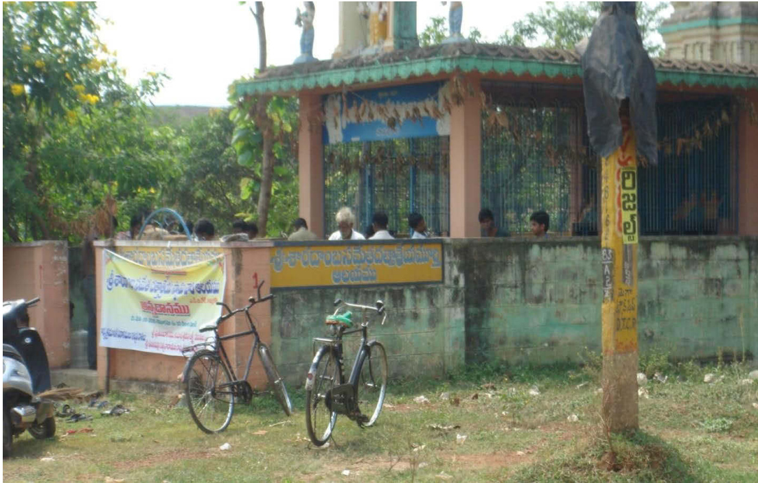
CPRs Sharadhamba Temple At Samarlakota Village Chainage 0+860
