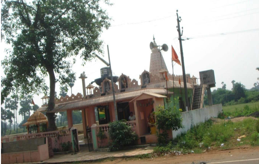
CPRs Sai Baba Temple At Vadiseleru Village Chainage 26+230
